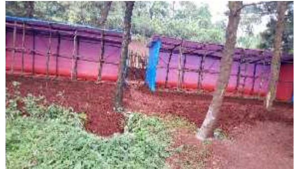
Picture 4: New toilets with 14 pits constructed at Cherba primary school, August,2018.
