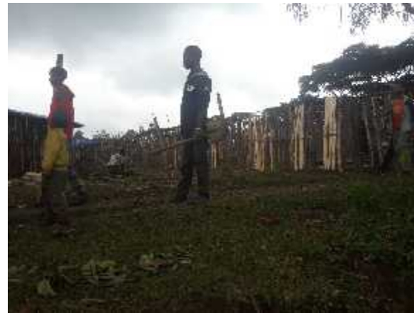
Picture 13: New temporary houses under construction by the returnee at Chirku kebele, 2018.
