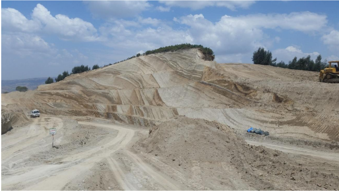
Plate: 5.3 slope cut and benches in volcanic ash road section around km 20
