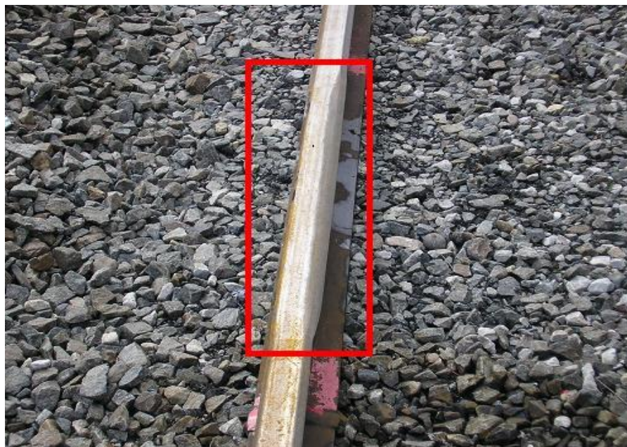
Shear Break Showing Dark Discoloration Identifying Defect Length
