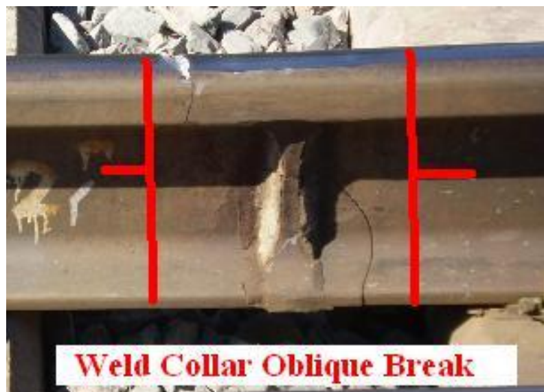
Thermite Weld Oblique Type Failure Originating in Web Area
