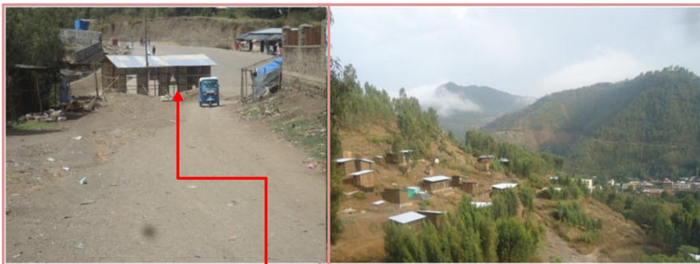
Figure 4.5 Illegal houses constructed on the road (left) and at Nitaf Dingay (right) (Source: Field survey, 2019)
