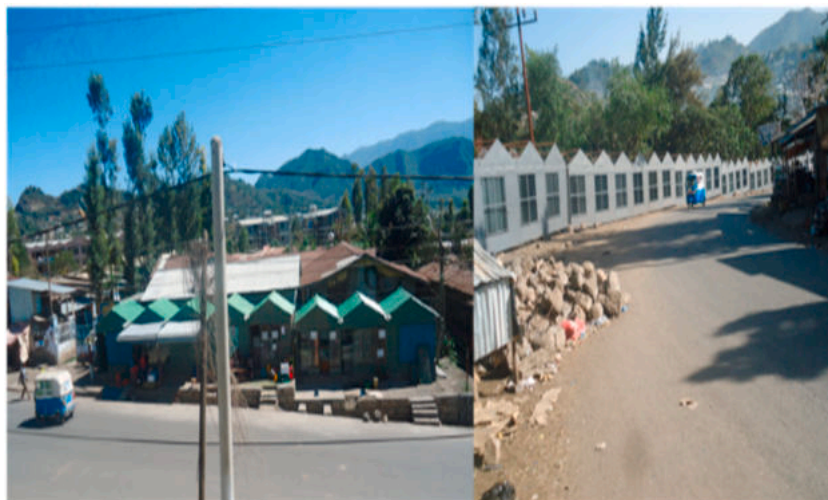
Fig. 6. Containers constructed illegally at the municipality's main gate (shown left) and along the steep road to the bus station (shown right). Photo by Author (2019).
