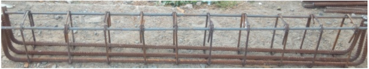
Figure 3-7 Reinforcement cage for CBM and CBC
