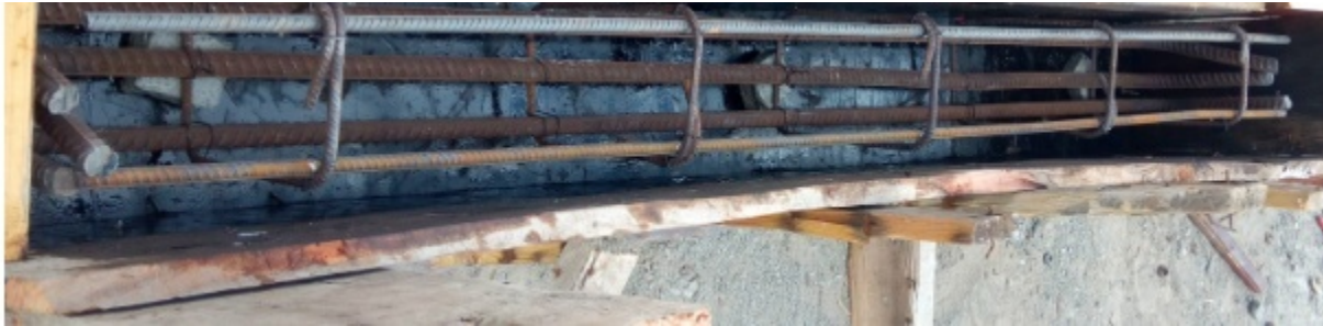
Figure 3-11 Installation of reinforcement cage into formwork
