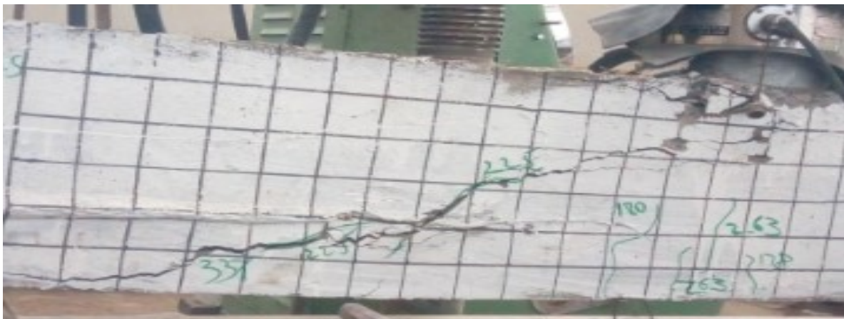
Figure 5-6 S50VF0.5%M after failure(close up view)
