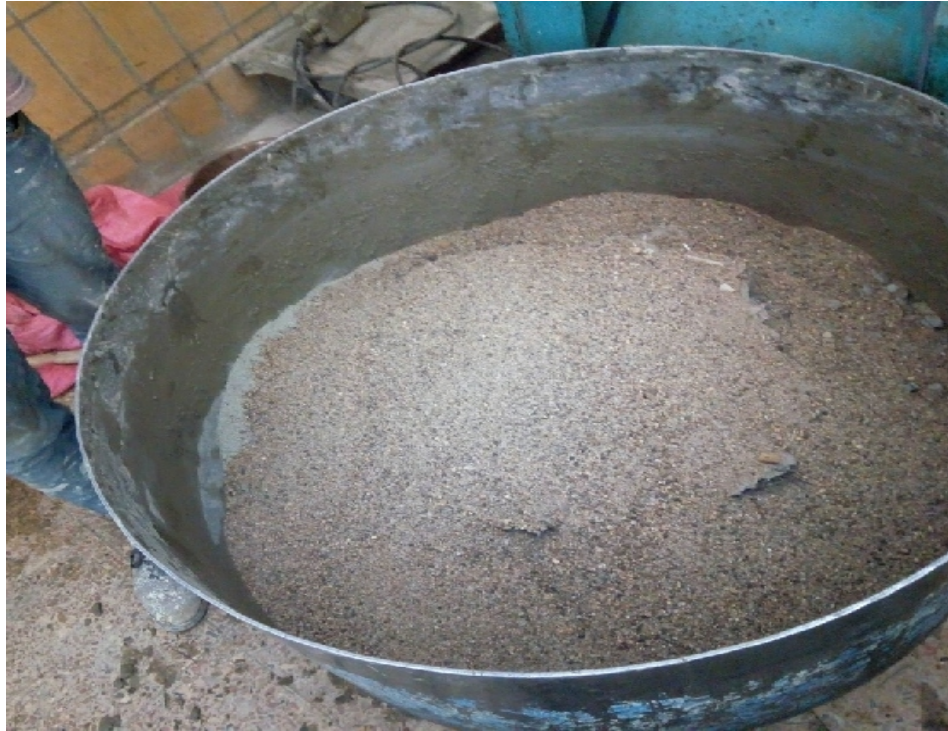
Figure 3-12 Adding concrete ingredients into the mixer
