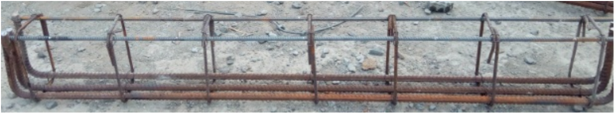
Figure3-8 Reinforcement cage for 50% increase shear spacing
