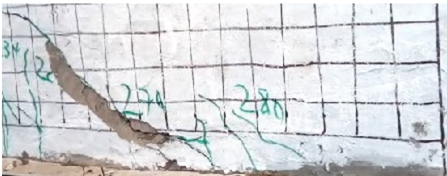
Figure 5-20 S100VF1.5%C after failure(close up view)
