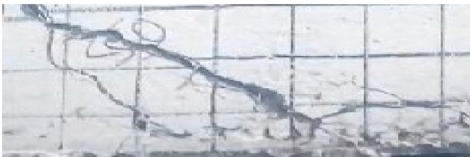
Figure 5-14 S50VF1.5%C after failure (close up view)
