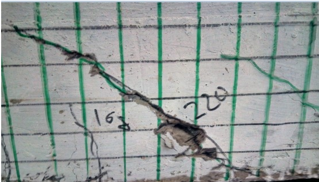
Figure 5-18 S100VF1%C after failure (close up view)
