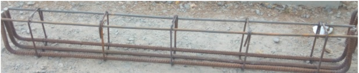
Figure 3-9 Reinforcement cage for 100% increase shear spacing
