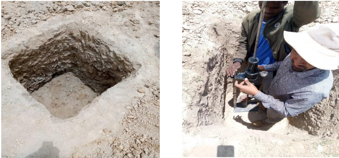
Figure 3-4: Excavated Test Pits
