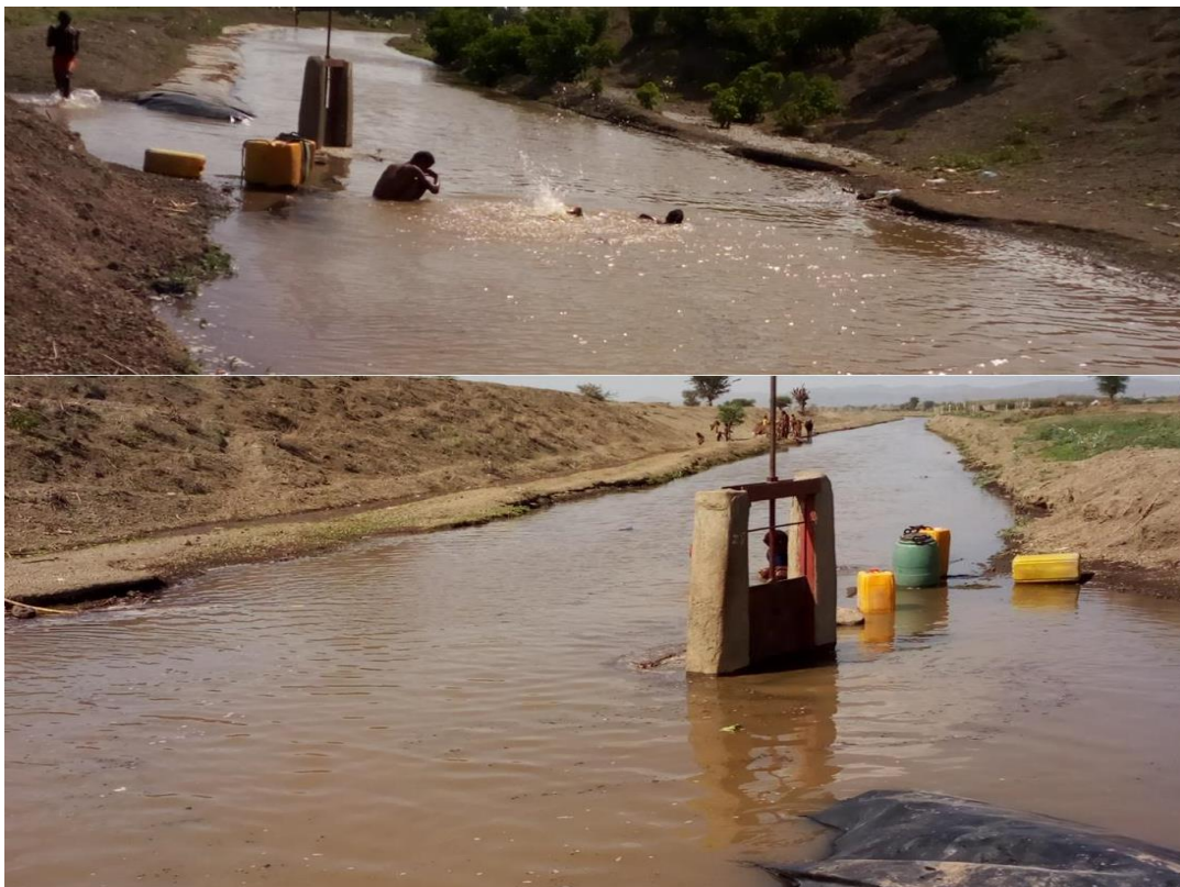
Figure 7-3: Excessive canal discharge in February, 2018
