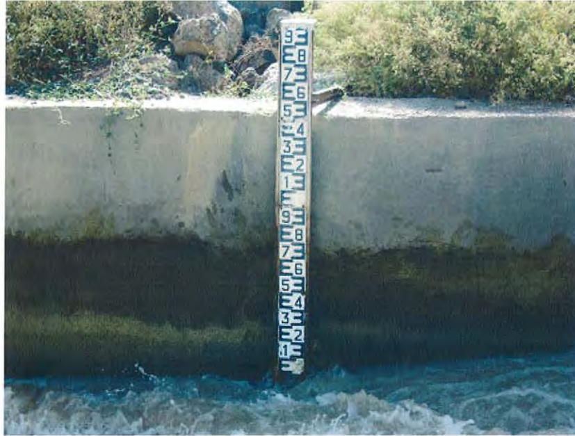
Figure 10: Water measuring at Head work
