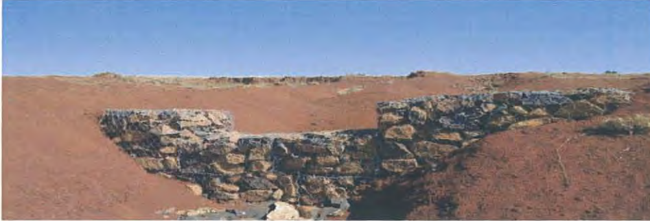
Figure 9: Gully rehabilitation by stone check dam (own photo at the field)
