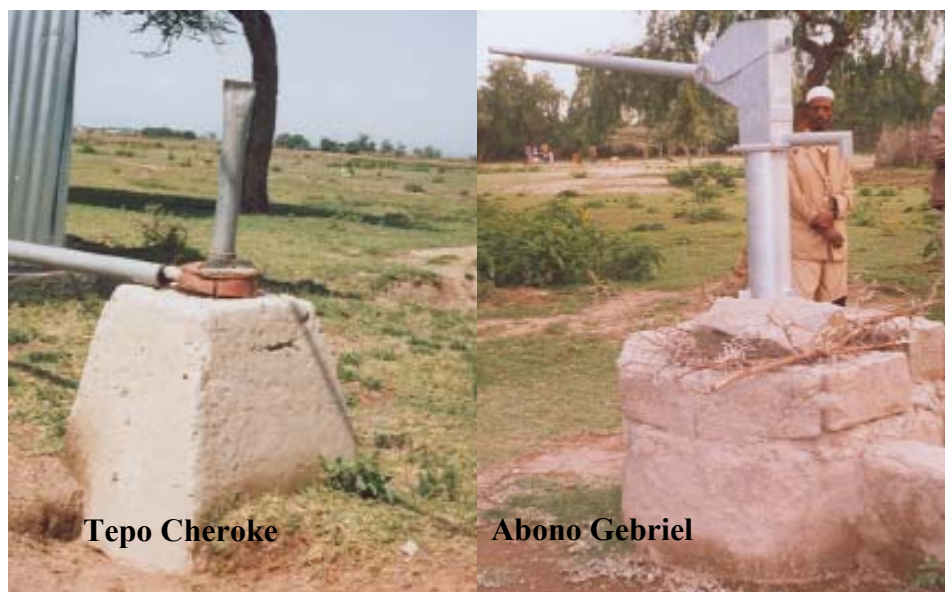
Figure 8-6: water schemes failed due to high fluoride concentration
