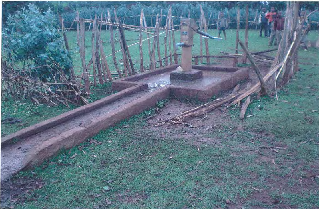
Figure: 4.5. Functional handpump without proper fencing and protection, Gowadamo, Aliwono site
