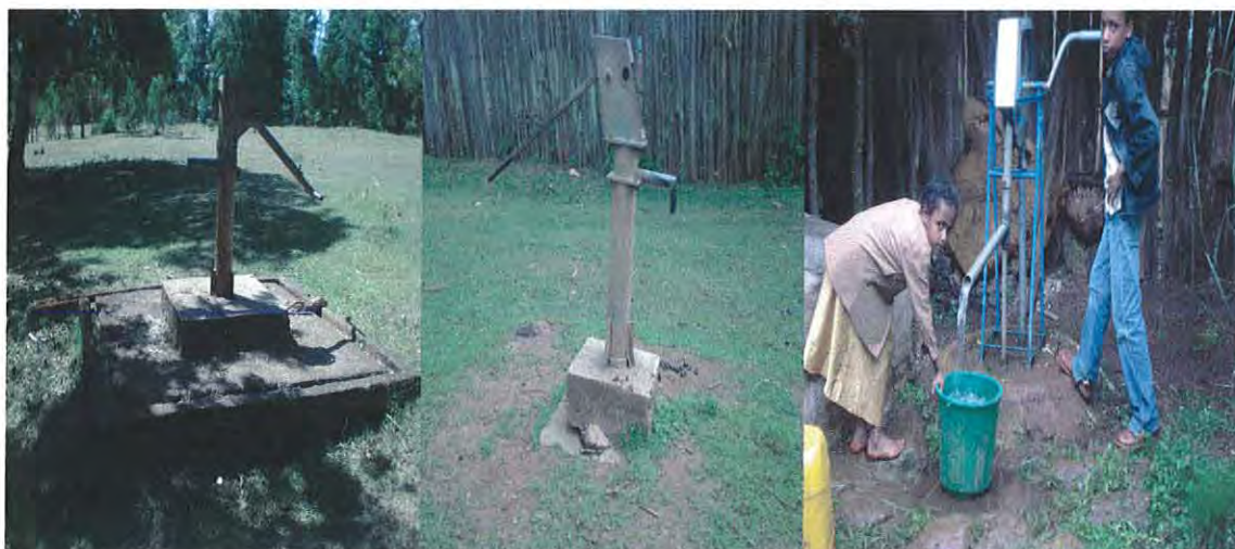
Fig: 4.2. Afridev (left), Indian Mark II (middle) and Rope Pump (right) handpumps
