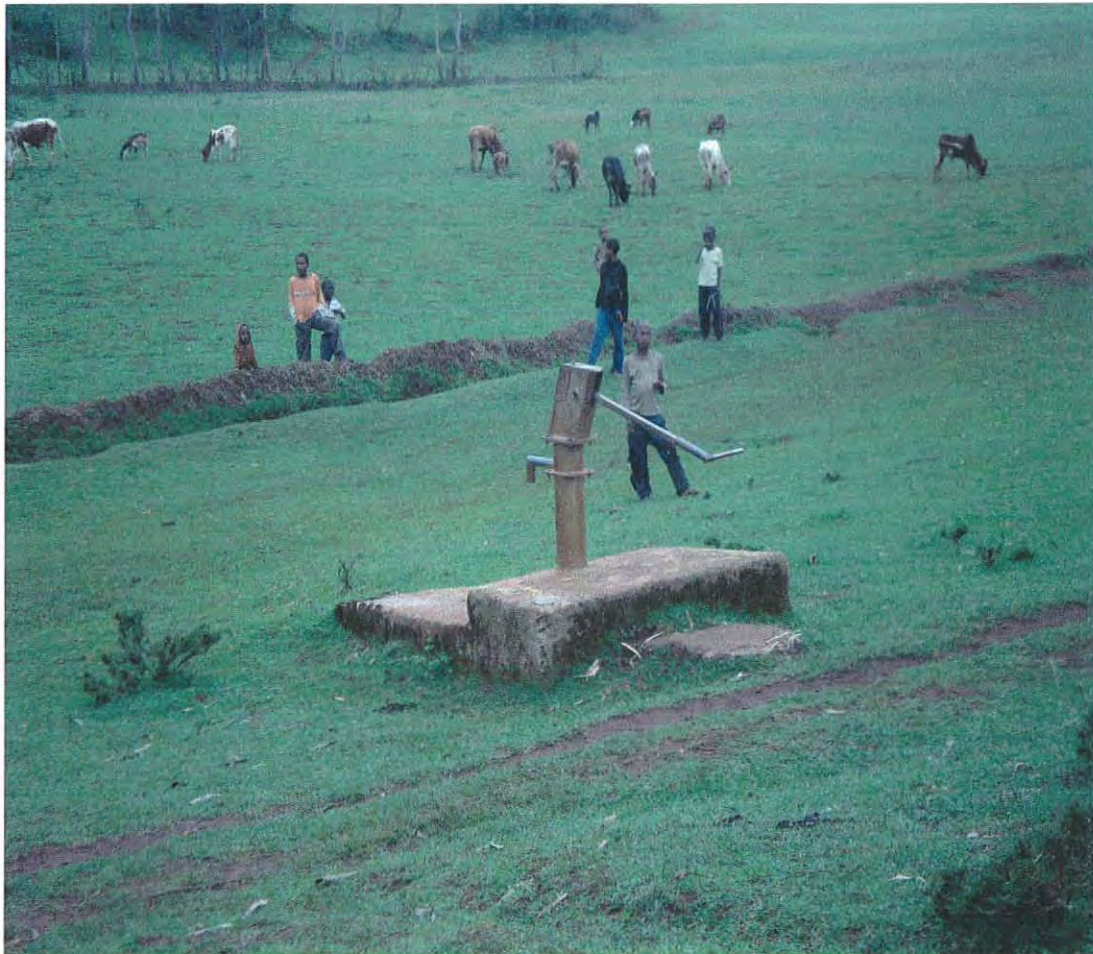
Figure: 4.7. Picture of abandoned handpump located/drilled in marshy ground, Gowadamo PA.
