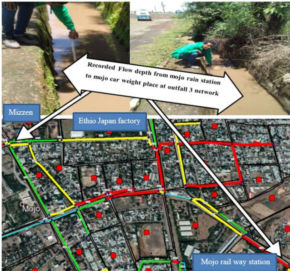
Figure 3-14: The recorded flow depth at site and drainage network
