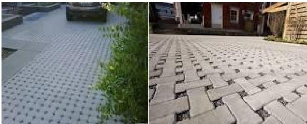
Figure 2-1: Permeable pavements method of structure view
