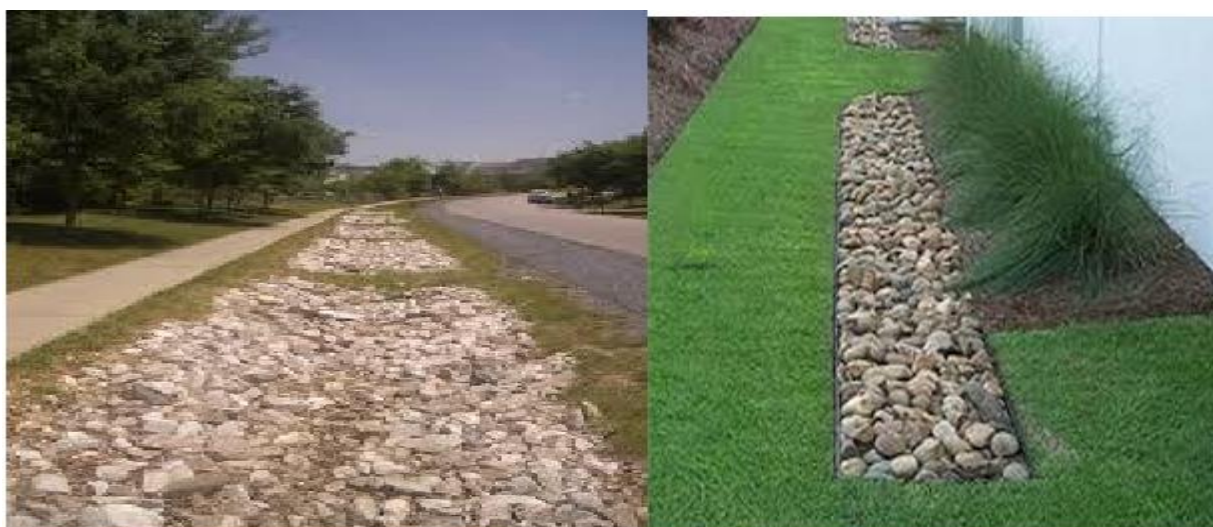
Figure 2-2: Infiltration trench structural view on side road
