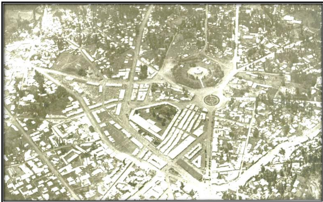
Figure 4 Aerial view of Arada before invasion in 1935; Source, (Fasil & Gerard, 2007)
