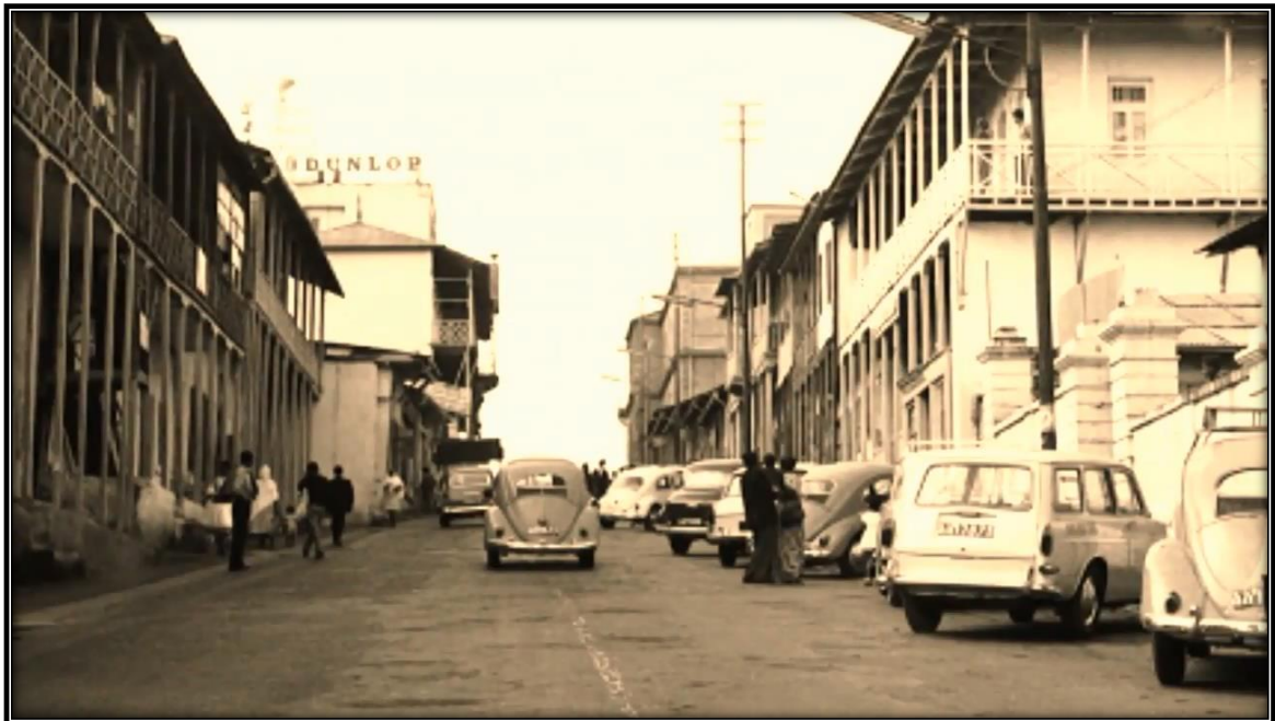
Figure 25 Characters of old buildings exists on Gandhi street.
