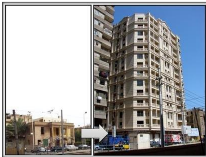
Figure 7 A small villa in the El-Raml area demolished to build a huge apartment building. (Source, The Arab Republic of Egypt, 2016)
