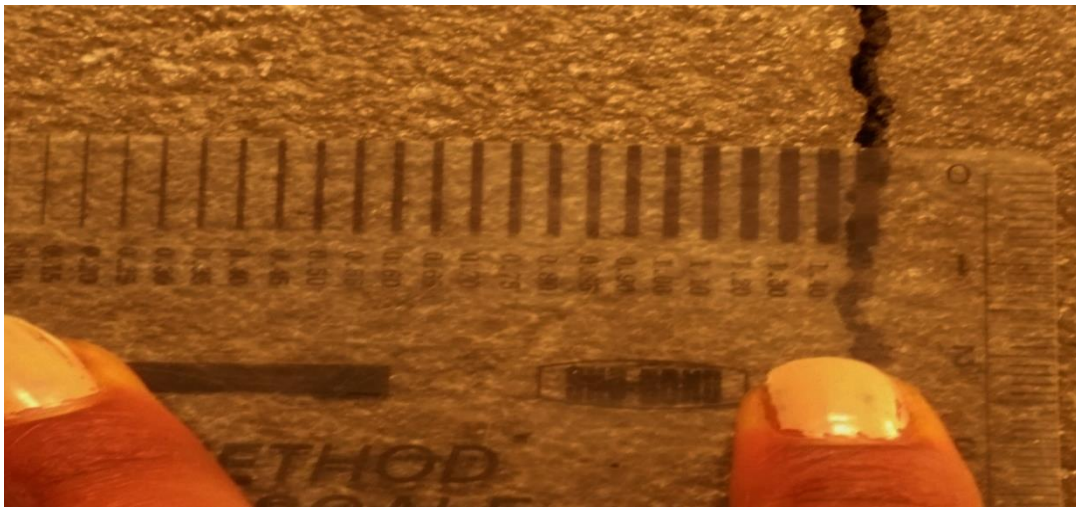
Figure 3-19 Manual measurements of crack width by Crack gauge card
