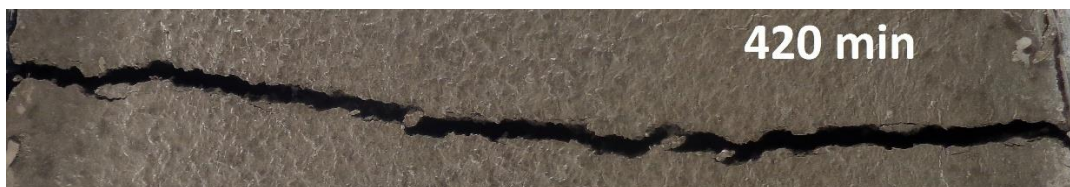
Figure 4-5 The propagated crack width of 0%
