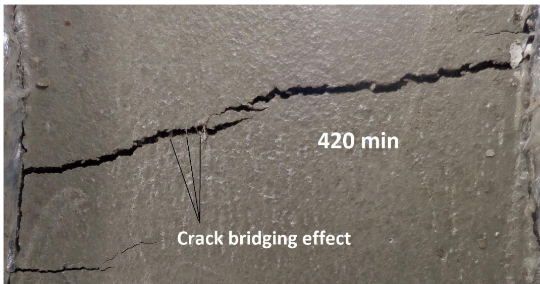
Figure 4-6 The propagated crack width of 0.0185%
