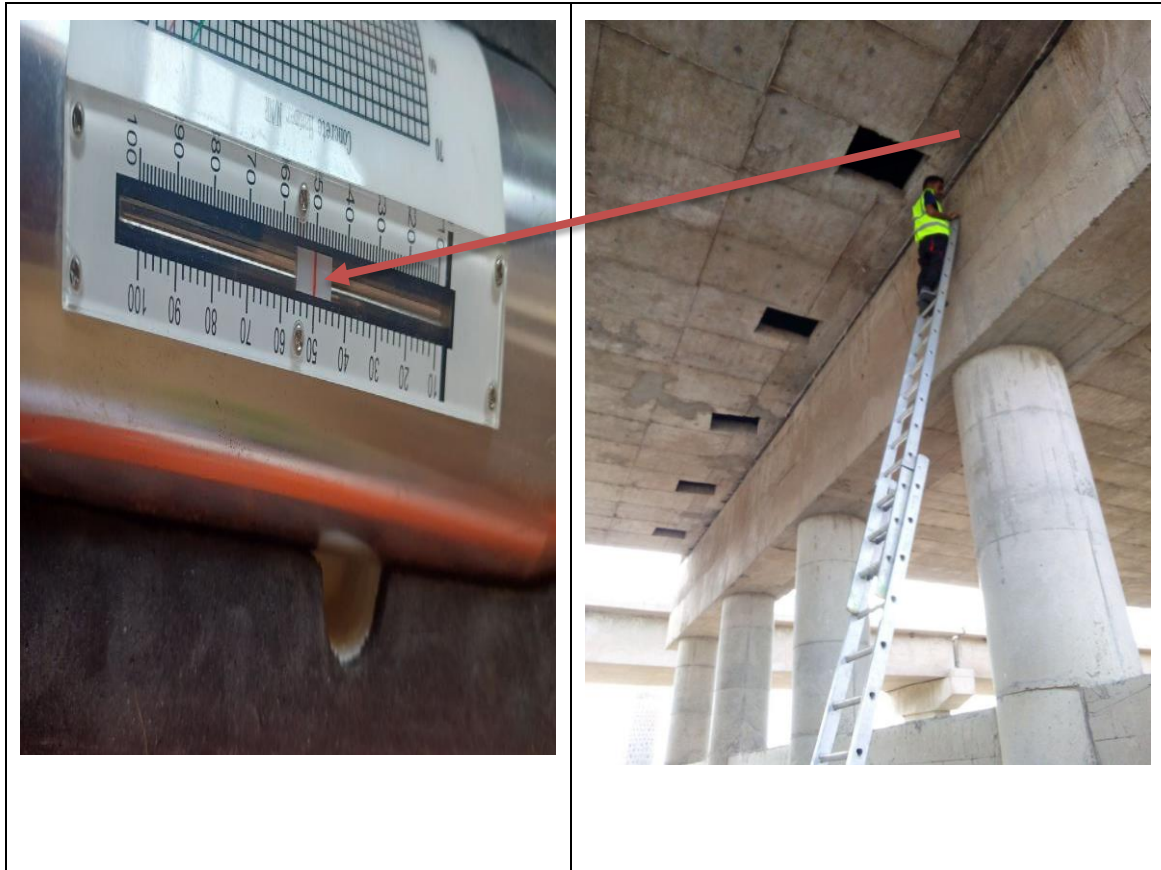
Figure 5-4 Sample of Conducting a Schmidt hammer sample on the Bottom Flange of the interior girder.
