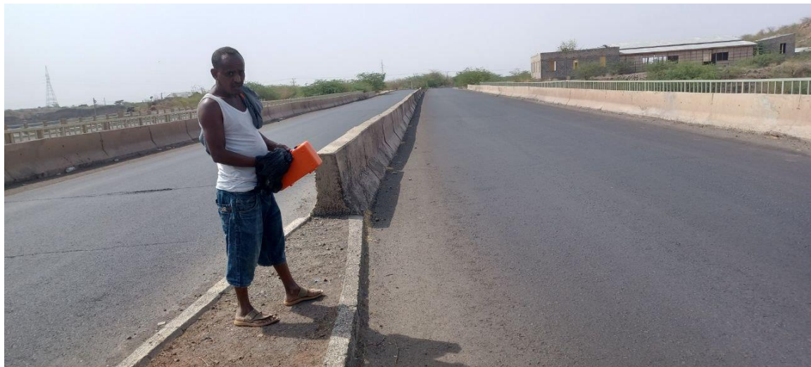
Figure 5-3 Existing Surface feature of Mille Bridge
