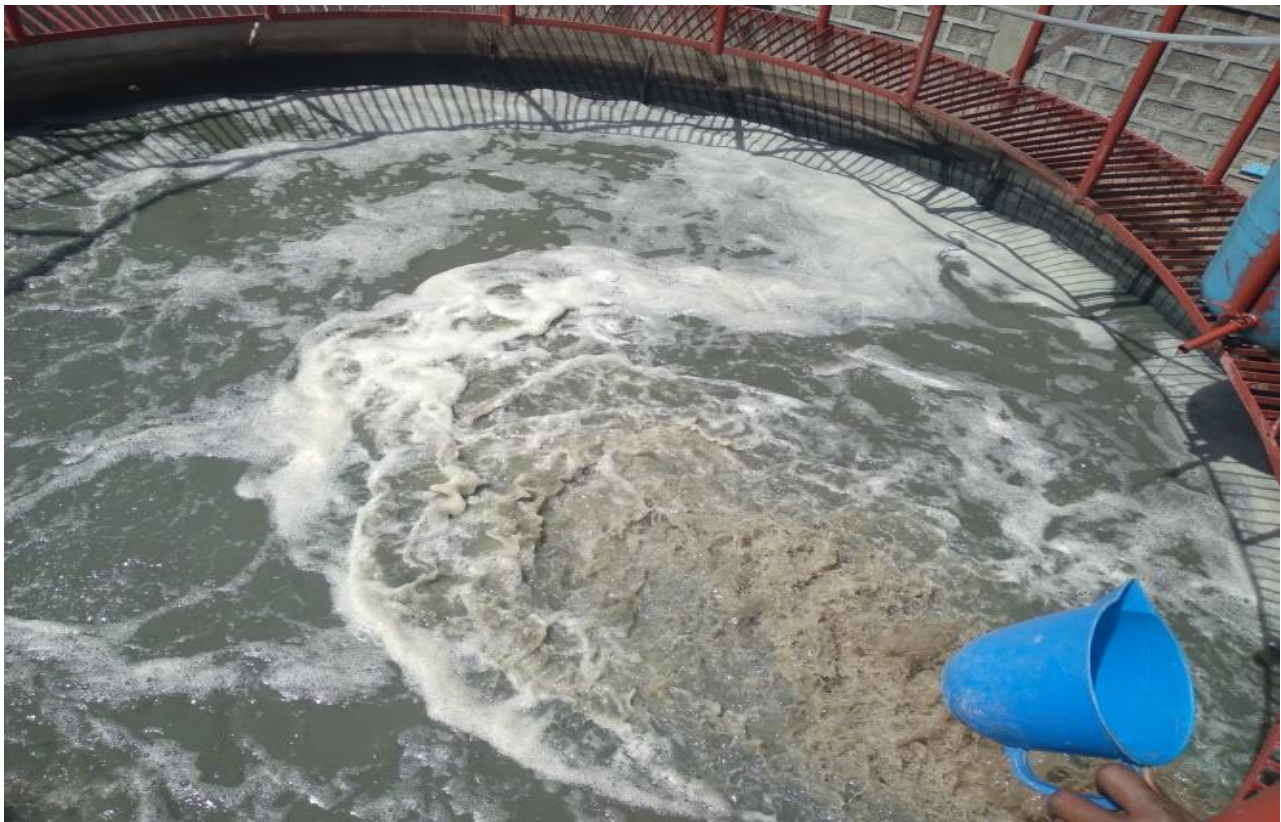
Figure 6: Sampling raw effluents from primary tanker
