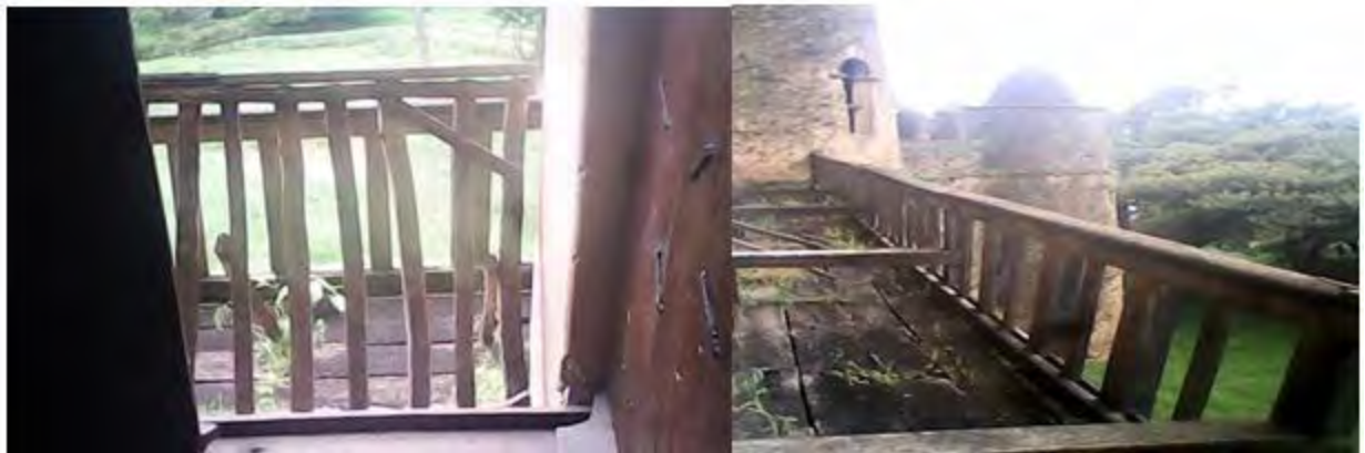
Figure 5: Restricted door which lead to Balcony (Source: Eskinder Desta)
