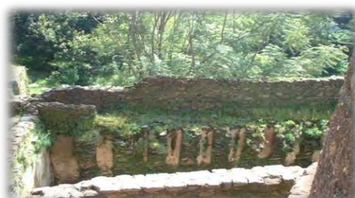
Figure 2: Buildings in deplorable state
