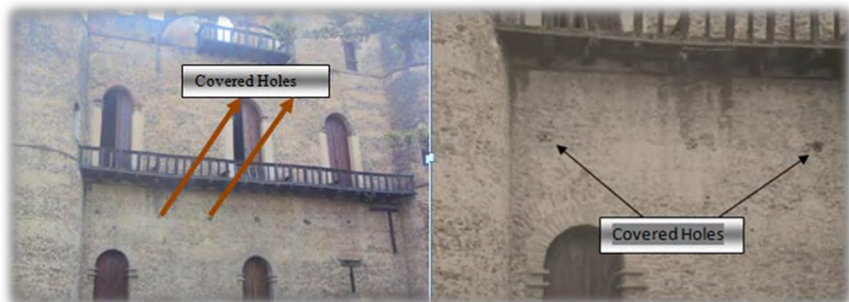
Figure 18: Covered holes for the wooden beams in the main Castel.
