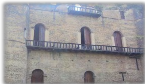
Figure 1: Buildings in good condition
