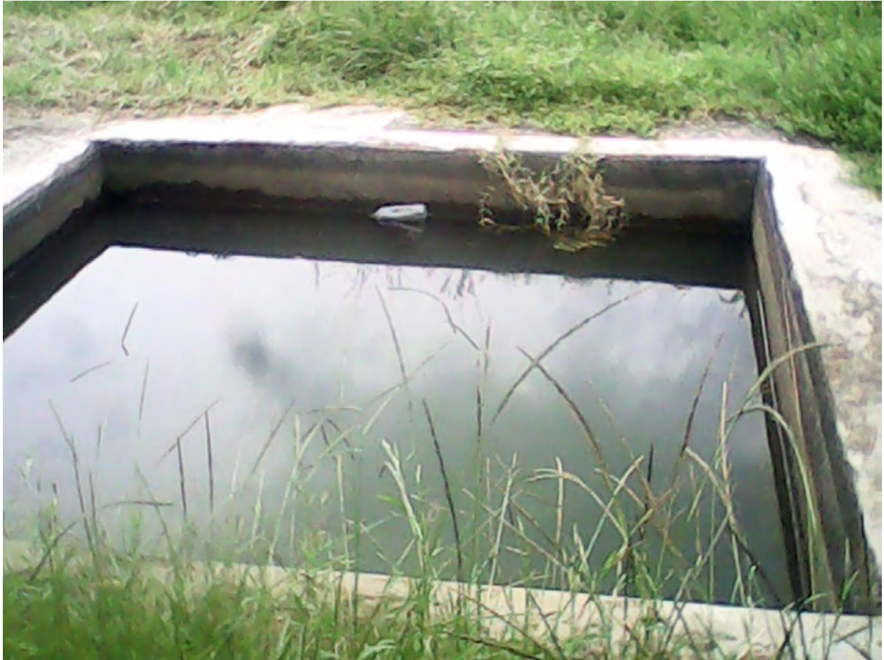
Figure 6: Hydration Pond in Fasil Ghibbi Palace Restoration Site (Source: Eskinder Desta)
