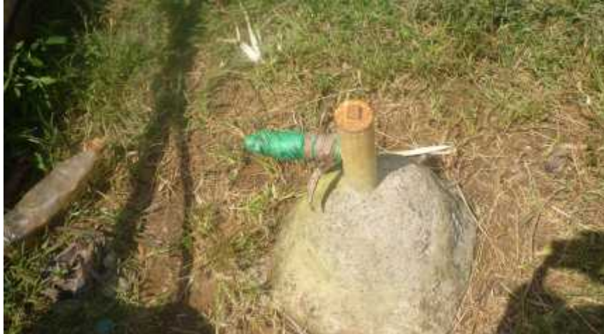
Figure 13. Dome cast high above ground surface
