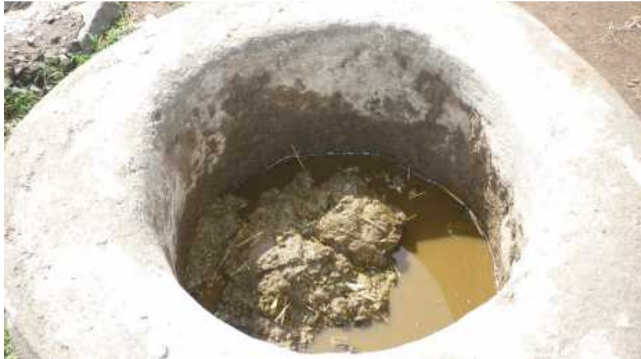
Figure 15. Dung mixed with chaffs ready for digester feeding
