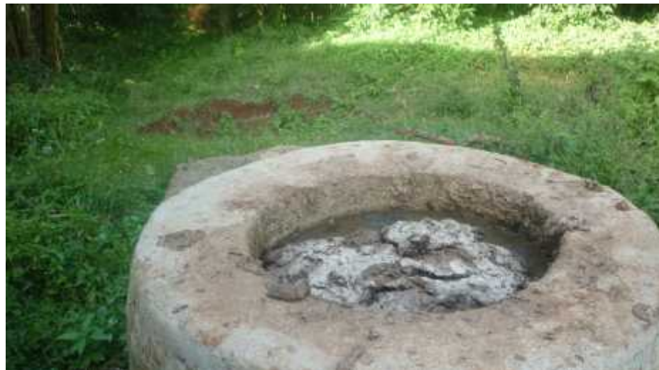
Figure 16. Dung stored in the inlet pit for later use has got dried
