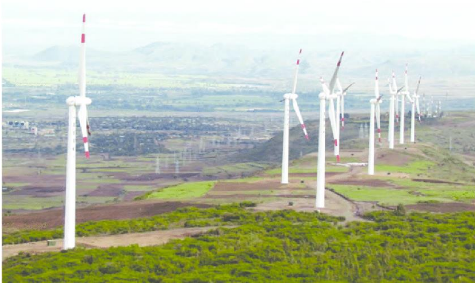
Figure 3: Adama I wind farm project (conventional wind turbine) A. MUKTAR [1]
