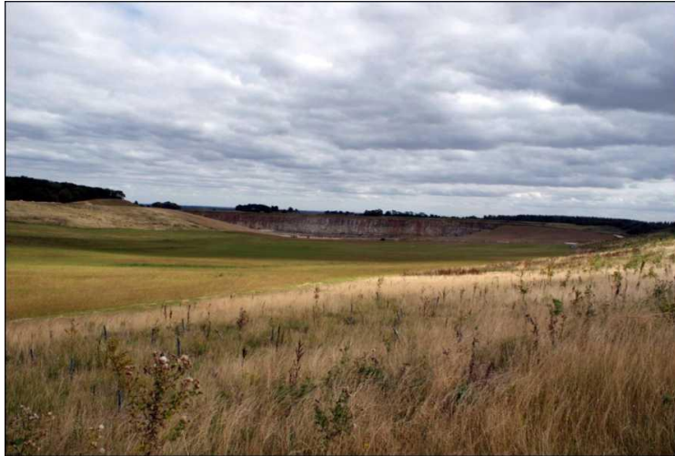
Plate 5 An example of rollover slopes being formed at the Hope Cement Works, Hope, Derbyshire, England. The technique was used in a progressive reclamation scheme to cover a number of benches where extraction has ceased.
