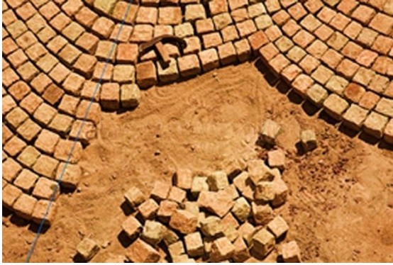
Plate 33 Paving roads and streets by Cobblestone
