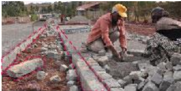
Plate 35 Defined road sides by curve stone
