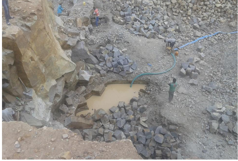
b) Stagnant water sucked by pump for channeling surface water
