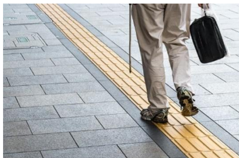
Tactile paving: provide a safer, more accessible environment for people who are visually impaired Source: https://www.allaboutvision.com
