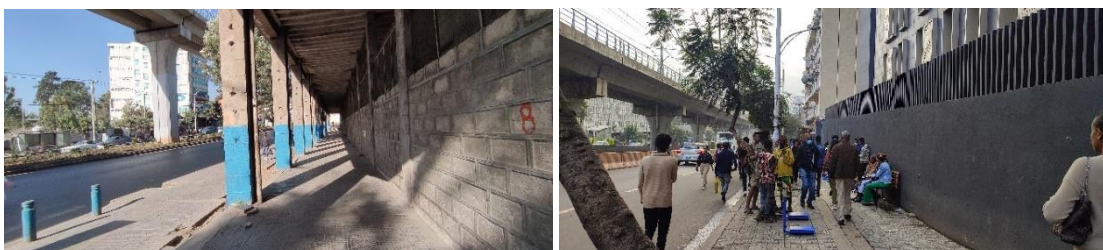
Figure 4.32Blind Street frontage impacted the activeness of the sidewalk.
