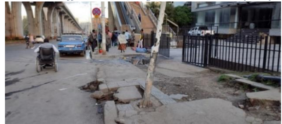
interrupted tactile pavements affecting visually impaired and non-wheelchair-friendly conditions
