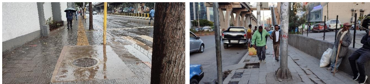
Figure 4.30 Obstructions and interruptions in the continuity of tactile pavement
