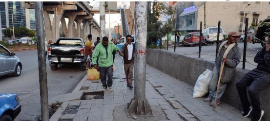
interrupted tactile pavements affecting visually impaired and non-wheelchair-friendly conditions
