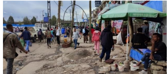
Unpaved and/or damaged pavement, holes, and related maintenance issues on sidewalks
