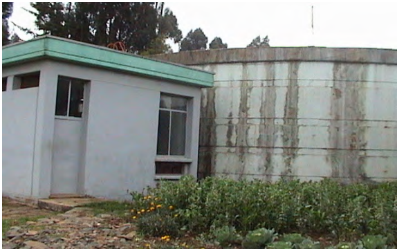
Figure 4-1 One of the Reservoirs at Rufael Rufael
