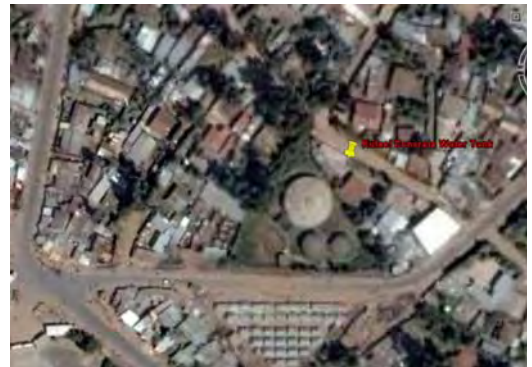
Figure 4-2 Areal view of Concrete Tanks at Rufael
