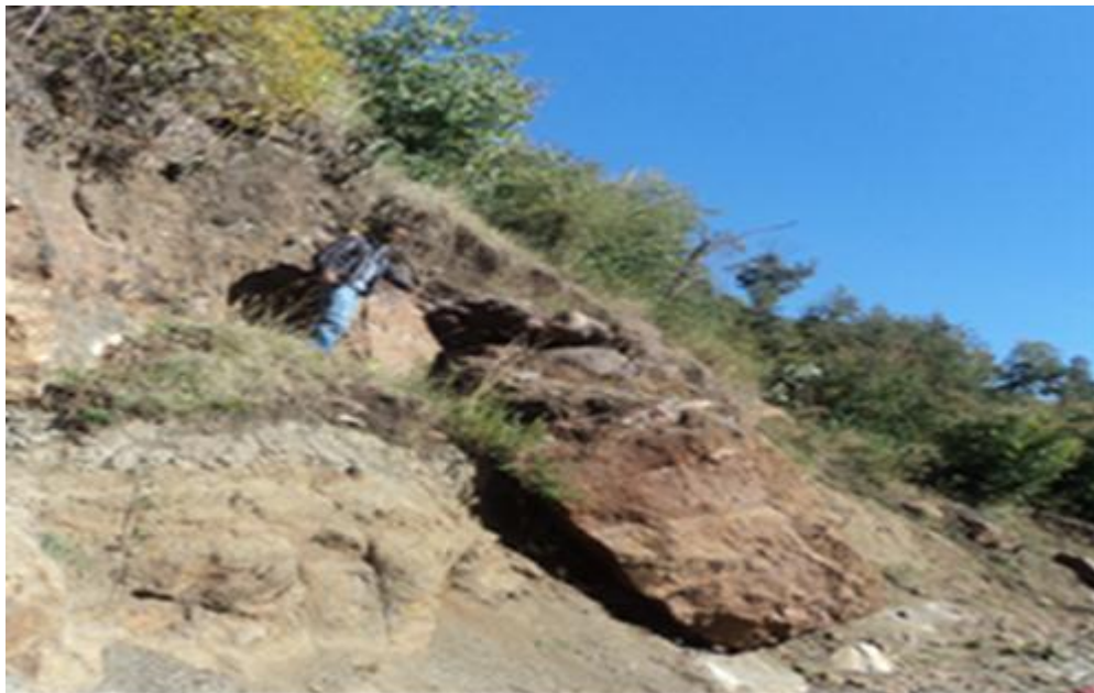
Figure 2.15 Rock slides at main road of study area
