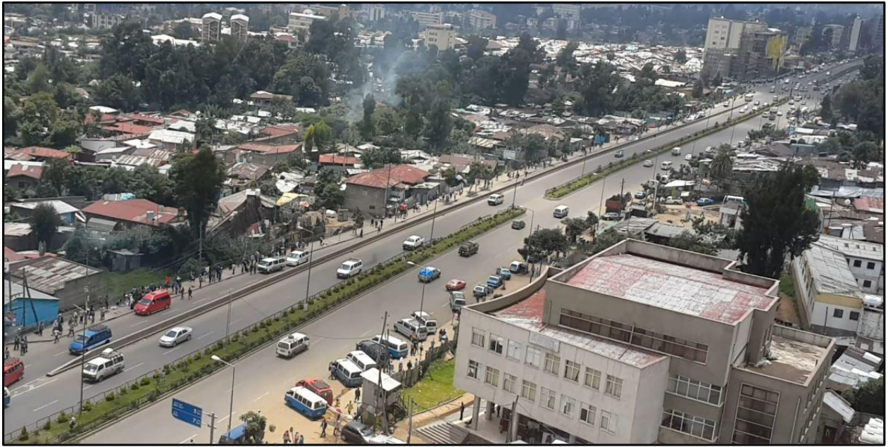
Figure 3.6: Video Camera View from Yeka Sub-city Administration Building (from the Building Right Side)
