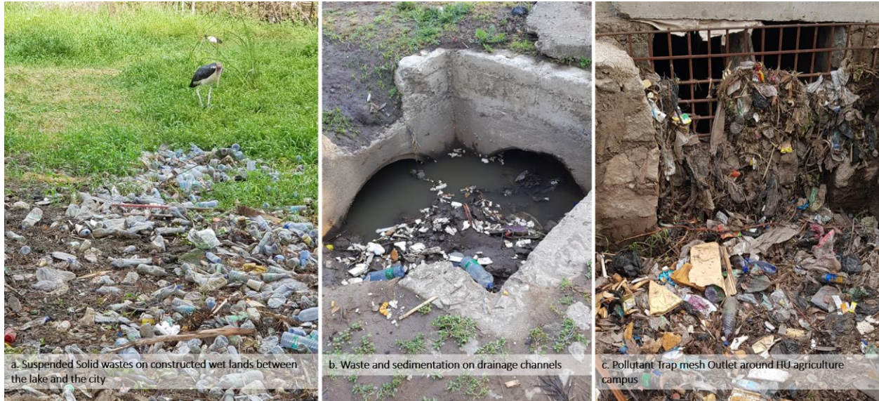
Figure 3.1-7 Picture showing pollutants on the surface and drainage outlets of the city to the lake. Source: Authors' site visit
