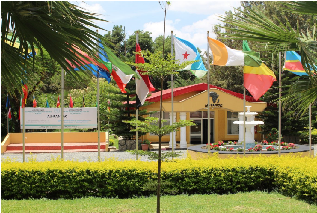
Figure 1: Administration office of AU-PANVAC
