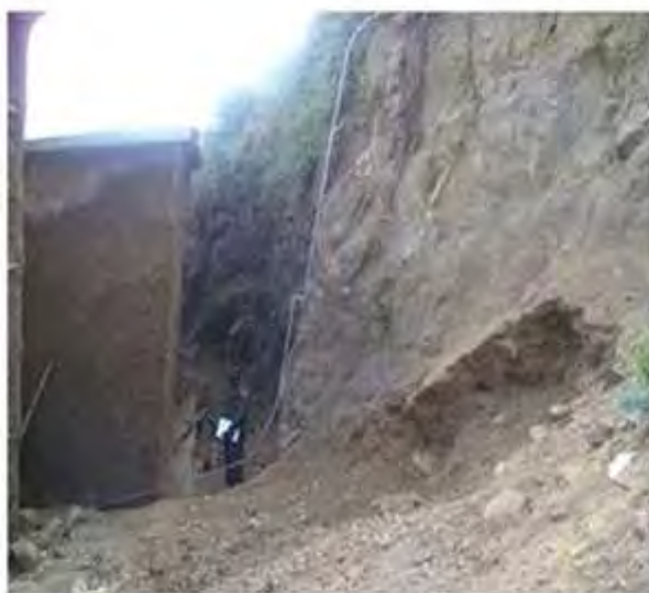
Plate 5.14 Slope cut for house construction in Mersa
