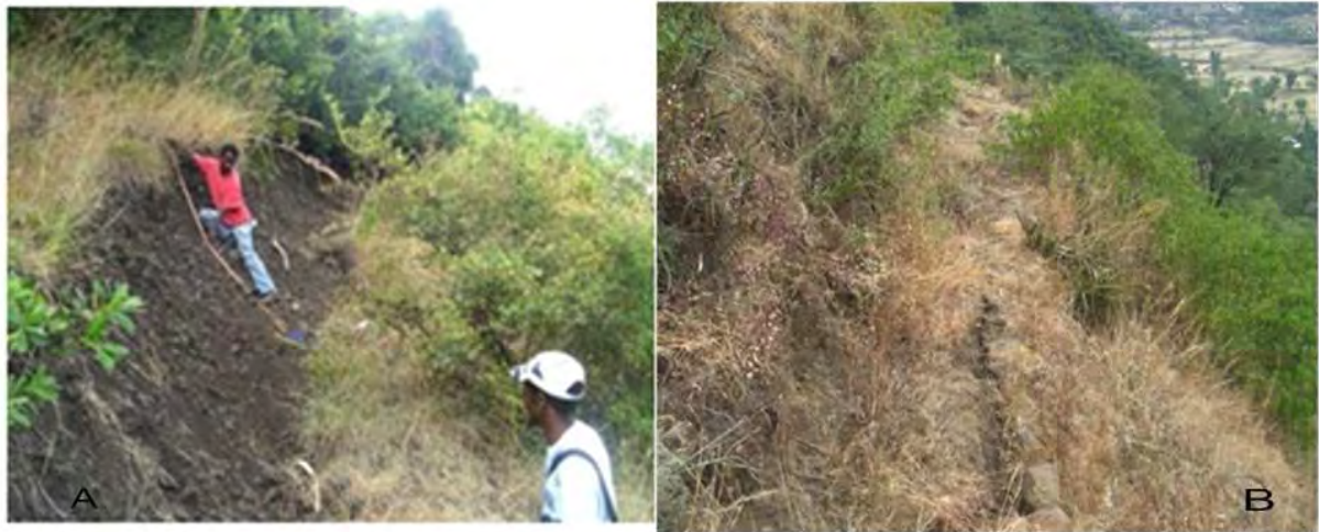
Plate 5.17 Displacement of cracked land (A) and tension crack (B) due to the 2010 Landslide Wurgessa
