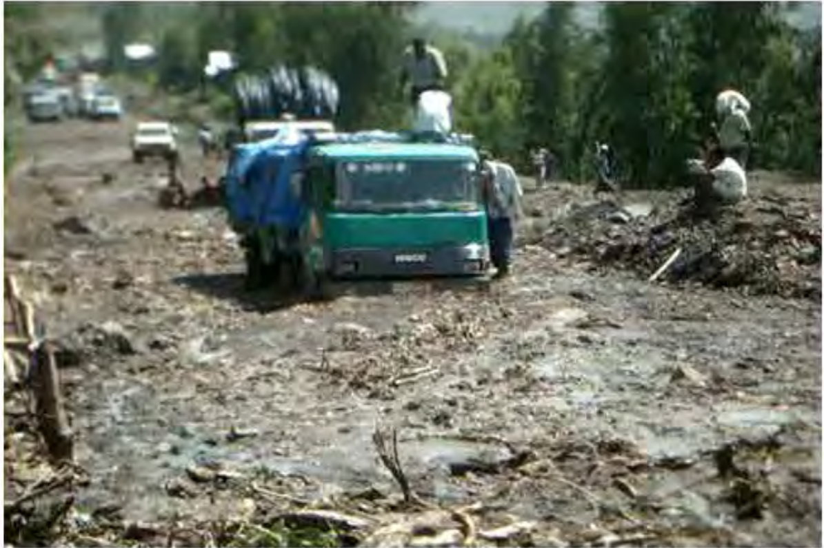
Plate 5.7 Debris flow due to Enqirt Wuha spring in August, 2010 (HWCO, 2010)
