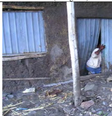
(h) Partially buried house by Debris flow in Wurgessa.
