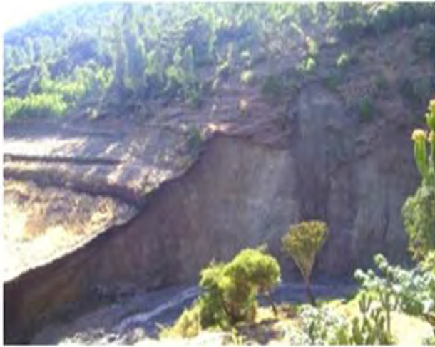
Plate 5.10 Slope toe erosion (Wurgessa)
