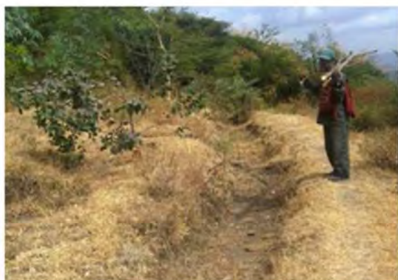
Plate 5.12 Drainage Ditches in the upper slope of the Main Landslide
