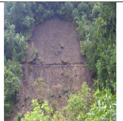
(i) Water pipeline has been damaged.
