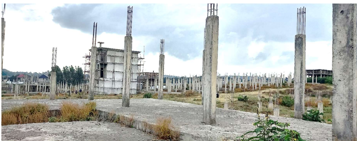
Figure 4-24 Unfinished Constructions Showing a lack of governmental supervision
