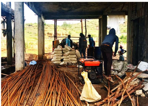
Constructions Using Generator due to absence of Electricity
