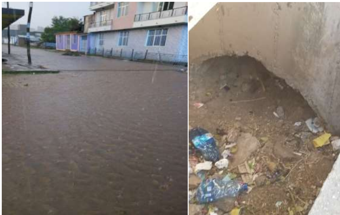
Figure 3.0.3 Flooding and silted drainage nodes
