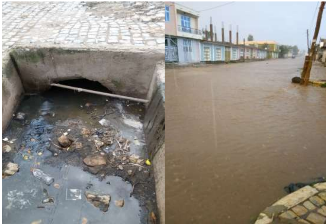
Figure 1-0.1 Silted Drainage and flooded the access road.
