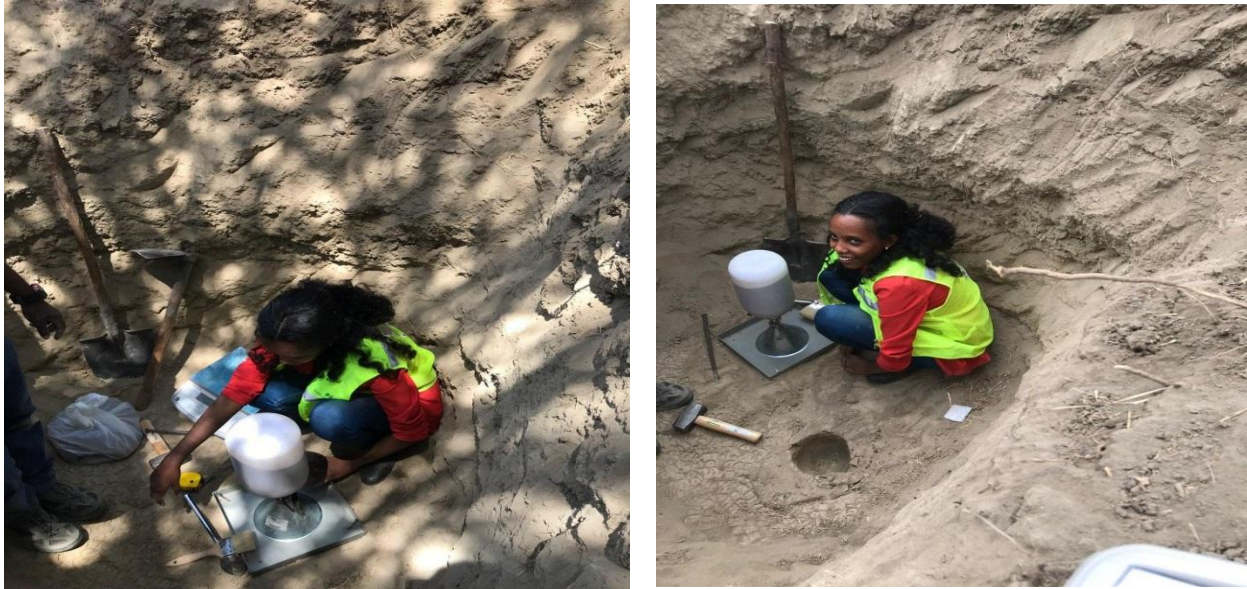
Picture 4. 4: Field density test using sand replacement method
