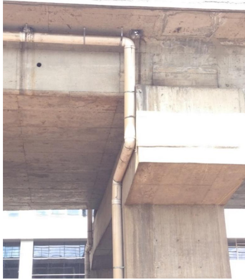
Figure 3.5: Saint Lideta Bridge
