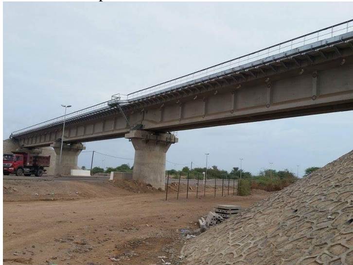
Figure 3.7: Route d'Arta bridge.
