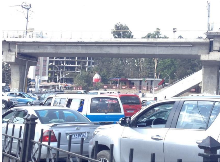
Figure 3.1: Saint Stefanos Bridge
