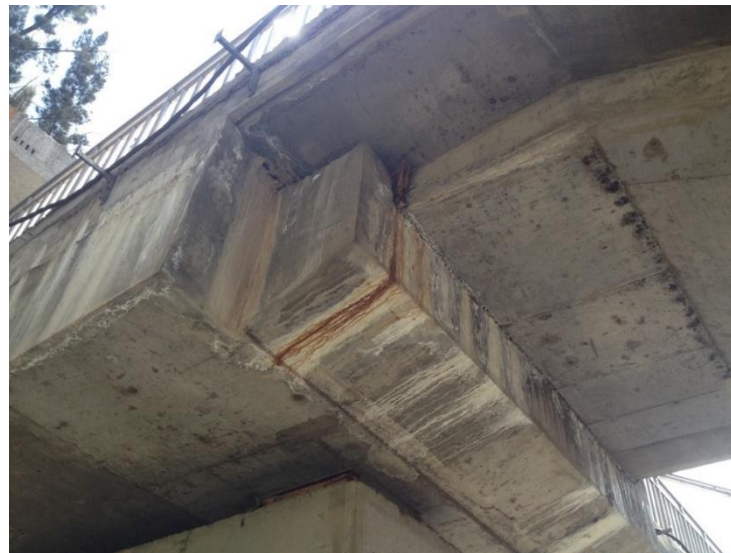
Figure 3.3: Tegbared Station Bridge
