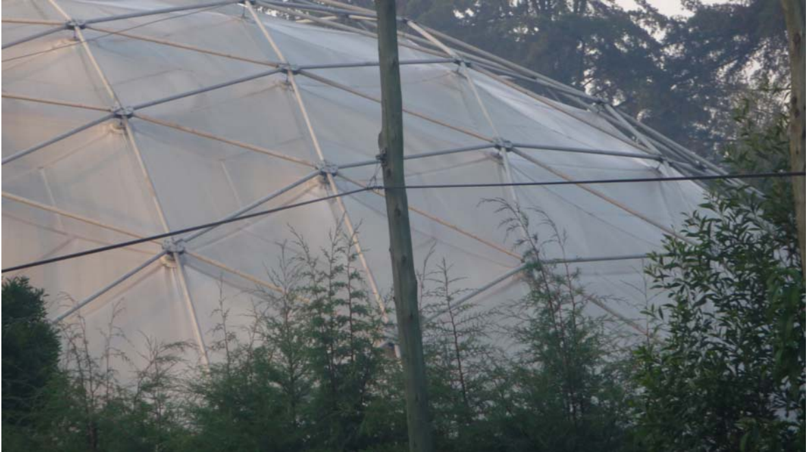
Figure 1.3 Single layer space frame of Ethiopian assembly hall
