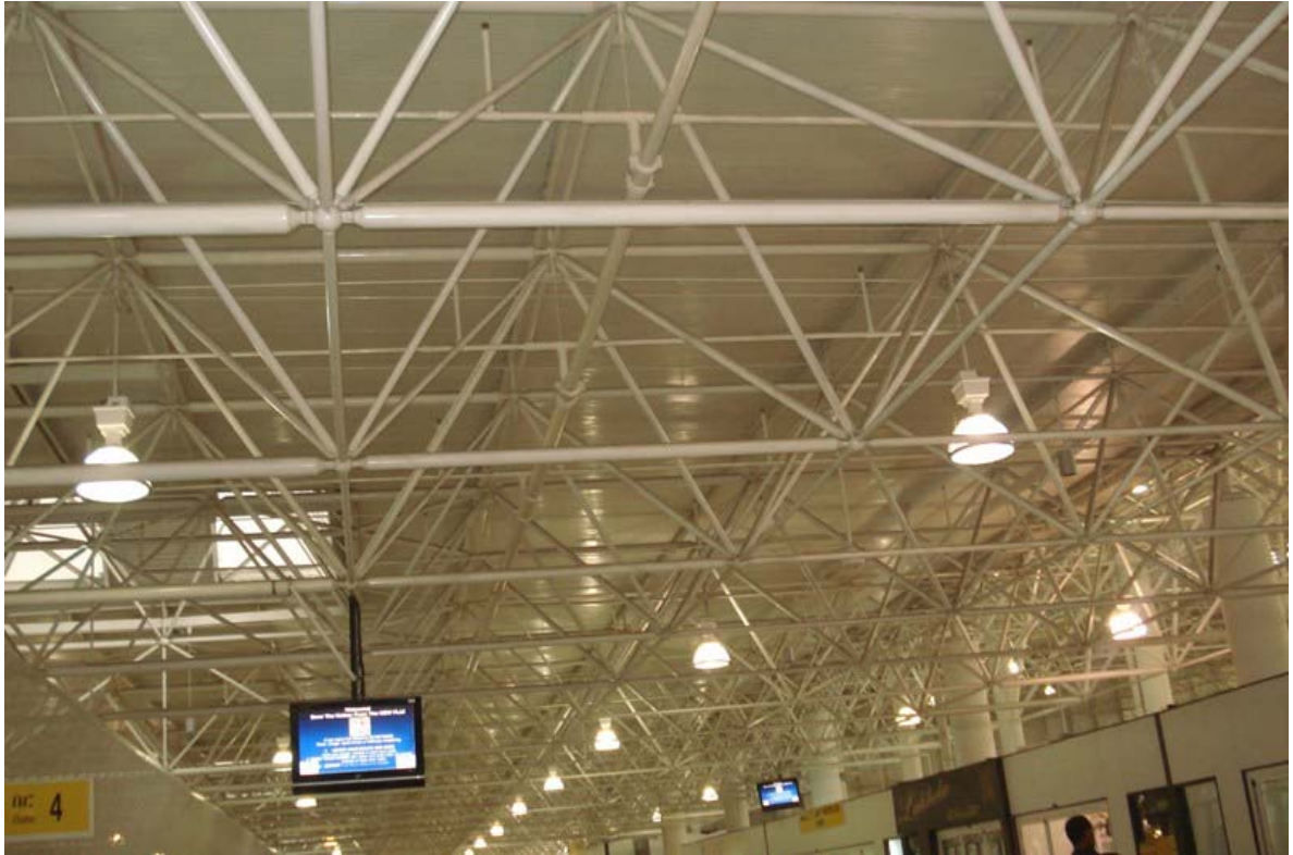
Fig 4.1 Orthogonal square pyramid space grids of AAIAEPT. (Photo by Abnet Abayneh, June 10, 2009, Addis Ababa)
