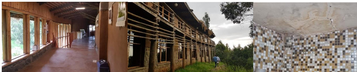
Figure 14: Naturally lighted and ventilated circulation (left), Wooden sun breakers (middle) and Dampness in the toilets (right)
