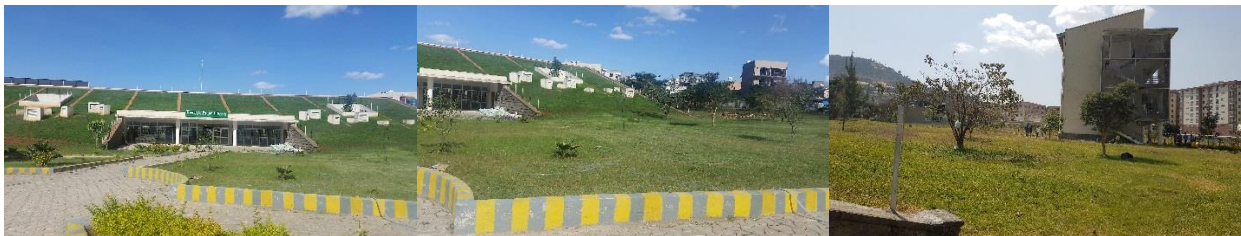
Figure 29: Green roof of the library and the surrounding green area (left to right)
