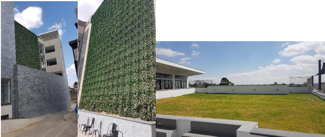
Figure 17: Green wall and Green roof of the building (from left to right)
