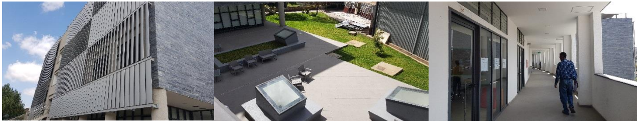
Figure 20: aluminum sun breakers (left), Skylight for the basement (middle) and naturally lighted and ventilated circulation (right)
