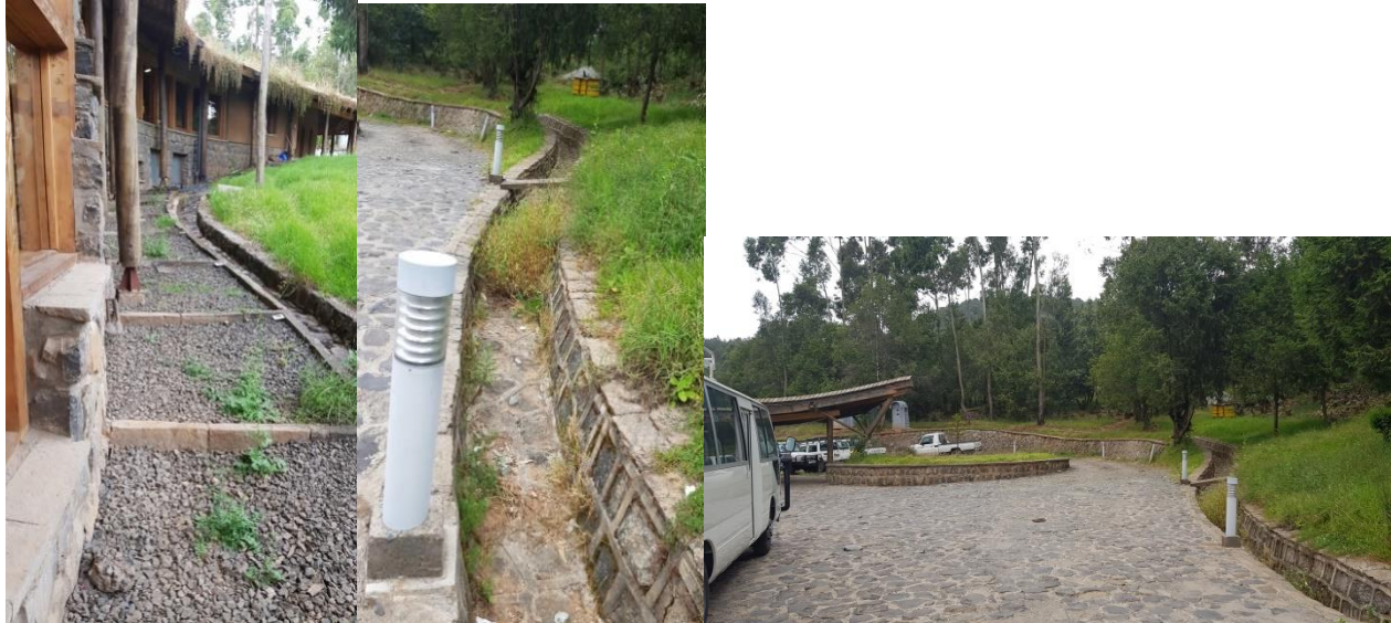
Figure 9: gravel infiltration trench (left), ditch channeling the stormwater to the surrounding green (middle), type of pavement (right)
