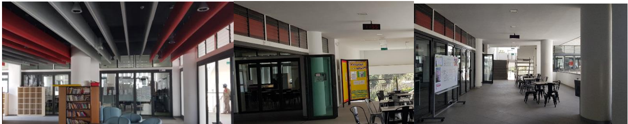
Figure 21: Acoustic panel fins (left), louvre windows and folding doors (middle) and outdoor recreational area in every floor (right)
