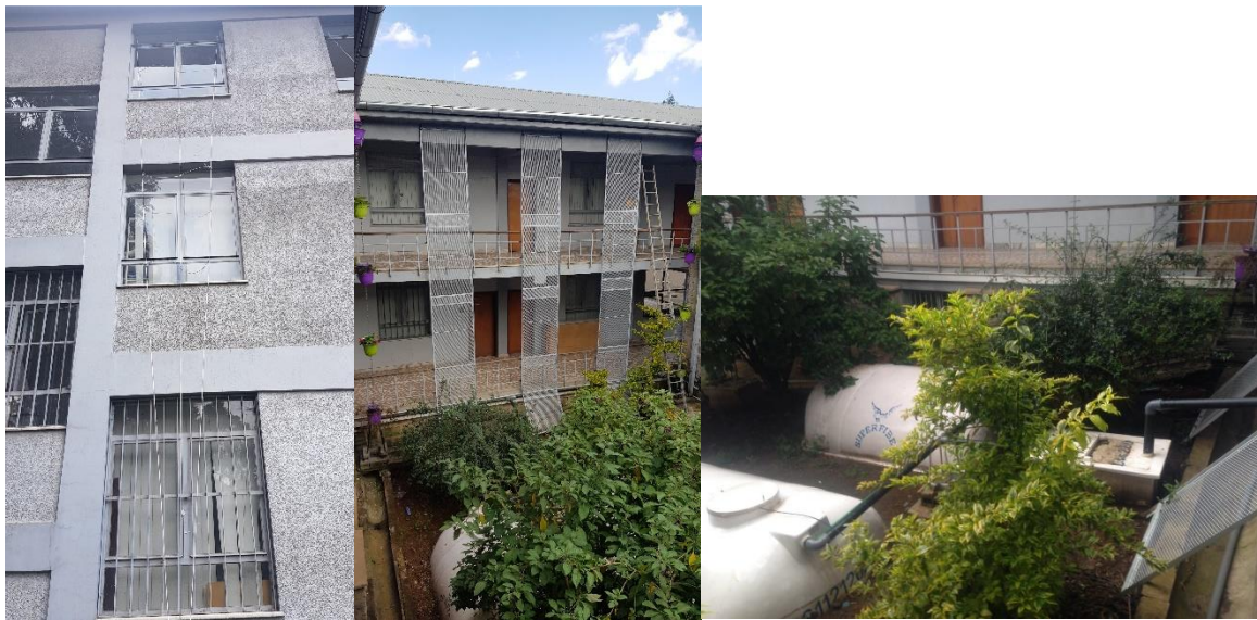
Figure 84: Constructed rope system vertical greenery (left), Constructed mesh system greenery (middle) and Fiber glass water storage for irrigation (right)
