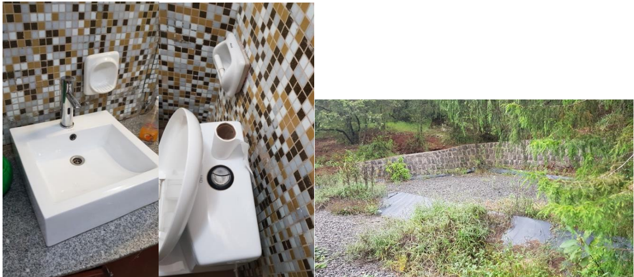
Figure 11: water efficient fixtures (left) and wastewater treatment (right)
