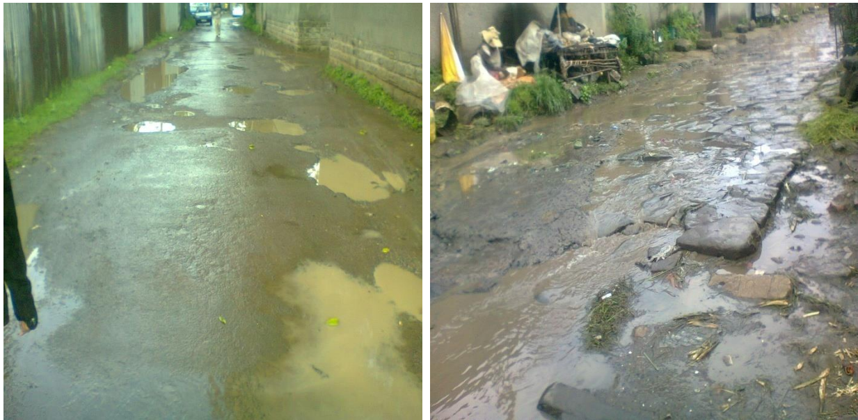
Figure 4.11 Roads without drainage network (source: Field survey July, 2012).
