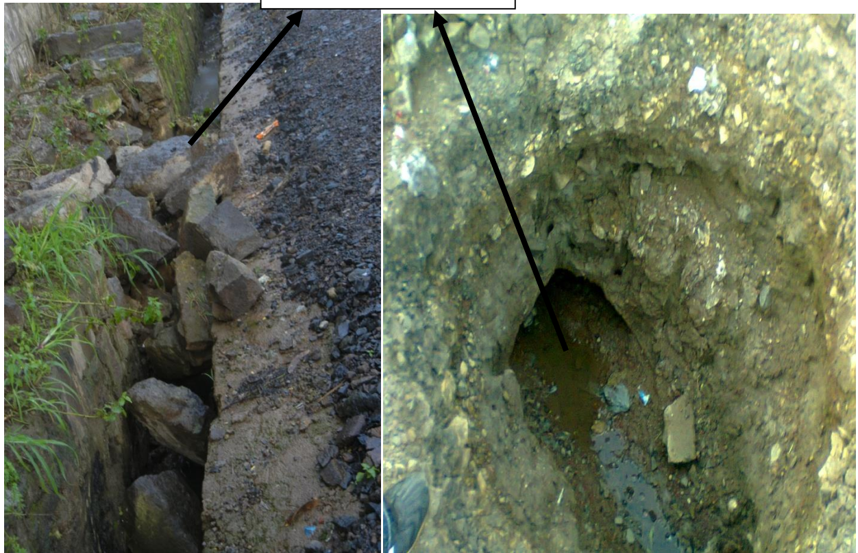
Damaged drainage lines
