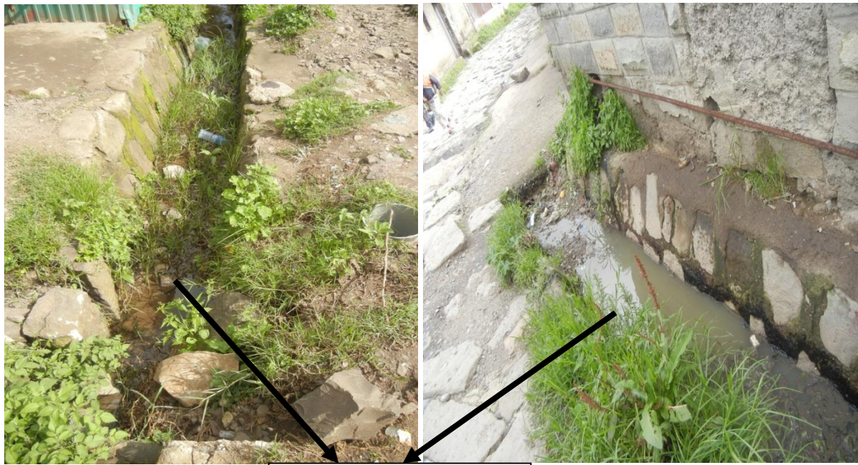
Damaged drainage lines
