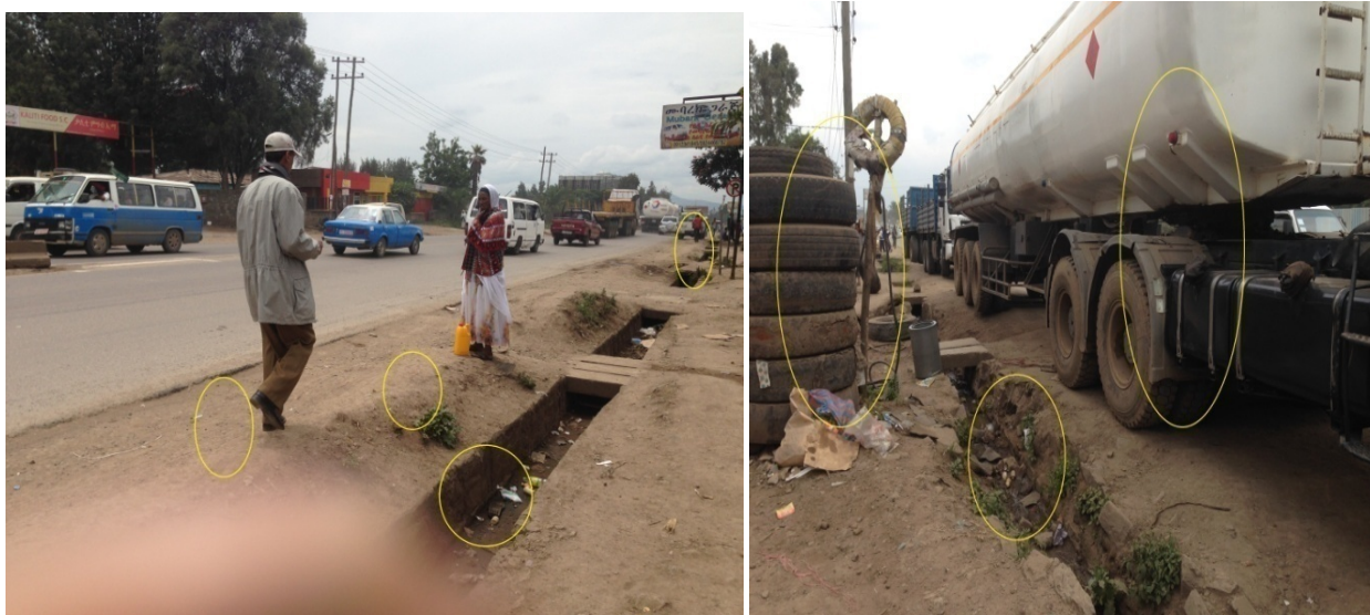
Figure 45. Photo. Improper drainages, Lack of pedestrian walkway and truck blocking sidewalk
