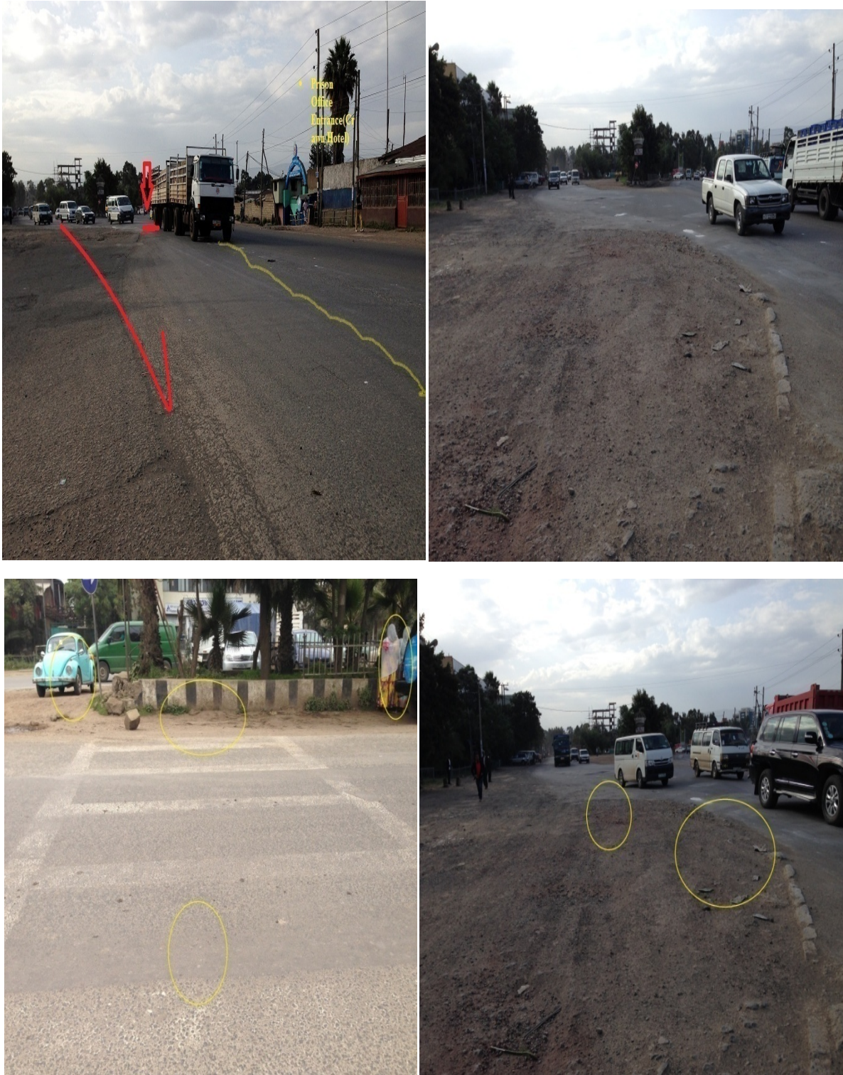
Figure 48. Photo. Faded and invisible pedestrian crossing markings, complete absence of lane marking (edge line, median markings, transverse), and no pedestrian walkway
