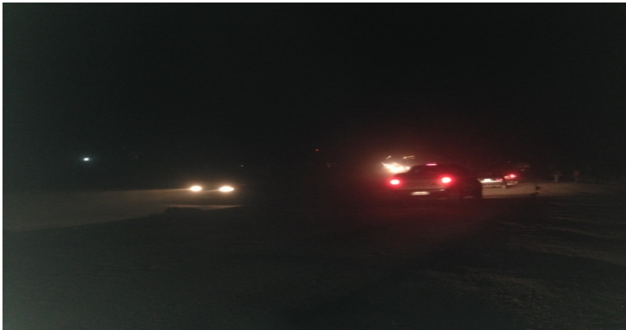
Figure 38.Photo. Night driving condition at Akaki- kaliti, that is absent of streetlights, pedestrian crossing lighting, generally no accessories for all road users.
