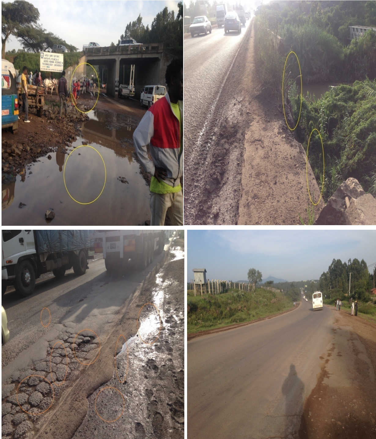
Figure 36.Photo. Pond of water at the Carriageway, complete absence of lane marking (edge line, median, and transverse markings), and lack of maintenance
