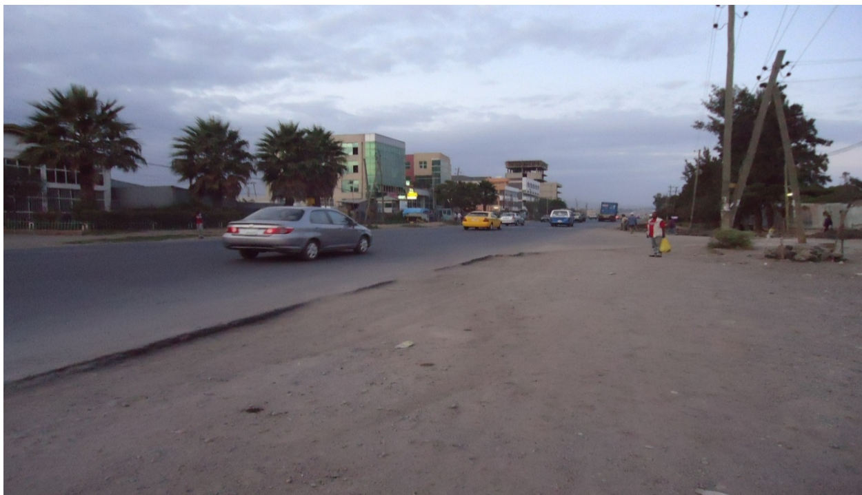
Figure 46. Photo. Complete absence of pedestrian crossing markings, lane marking (edge line, median markings, and transverse), and no pedestrian walkway
