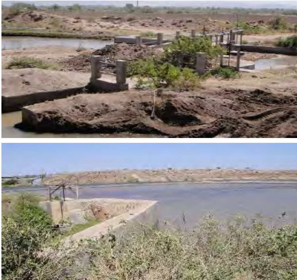
Figure 4.3 Pump station intake site (left) and Night service storage reservoir (Right)
