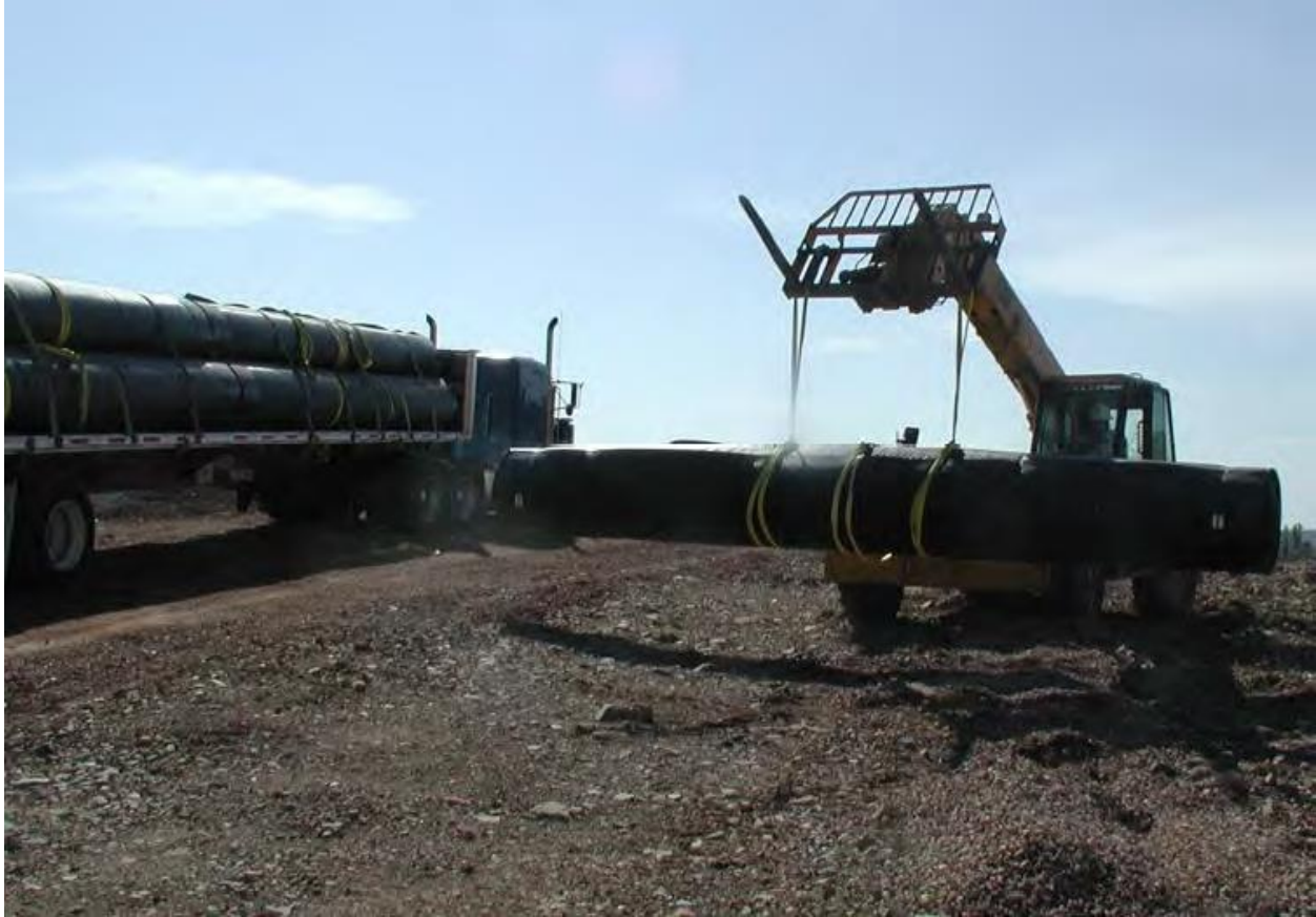
Figure 14: Photograph showing proper depositing of geotextile product rolls.
