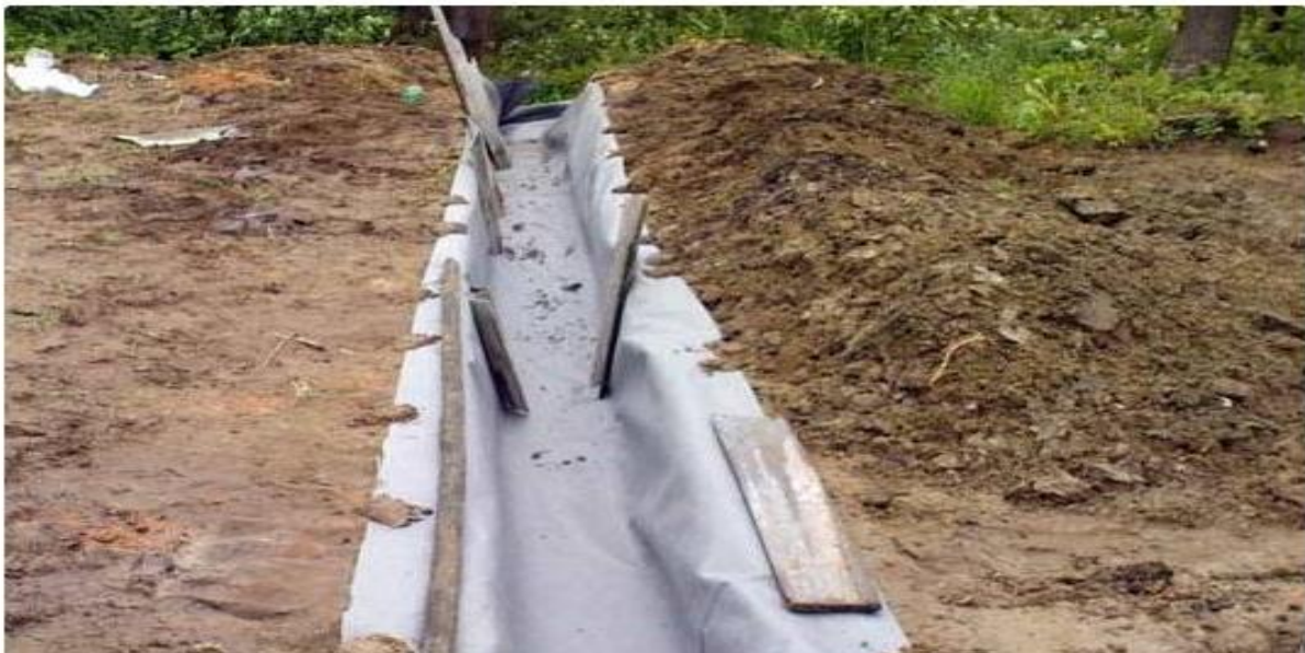
Figure 3: Geotextile use for drainage
