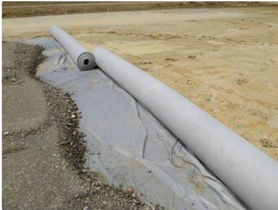
Figure 4: geotextile use as separation
