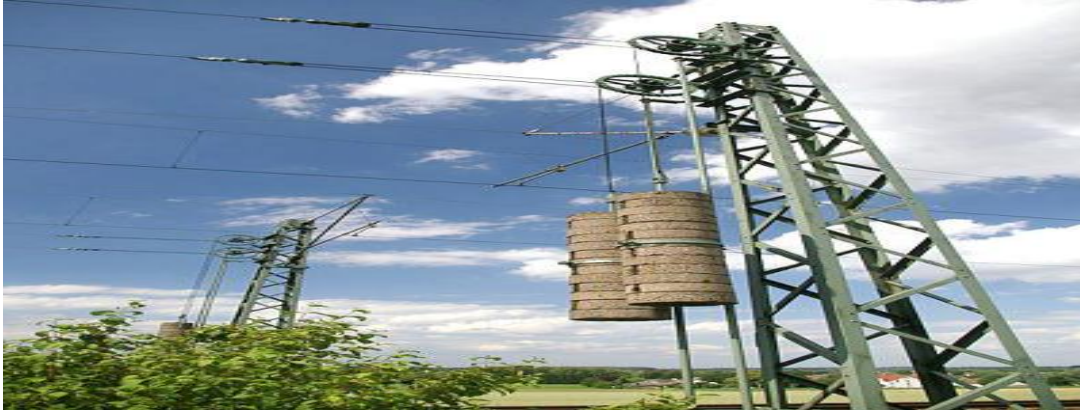
Figure 13: The photo shows the tensioning system of contact wire [12]
