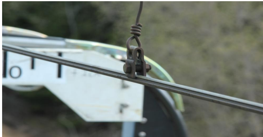
Figure 17: Dropper clamped onto the contact wire (Photo: Petter RøeNåvik). [8]
