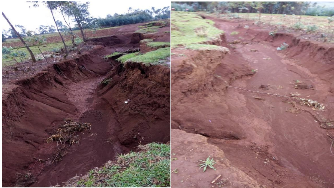
Fig.3 Gully erosion in Baka koricha kebele (Picture by Hundessa T.)
