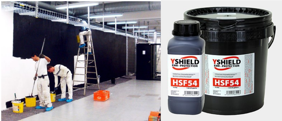
Figure 4: EMF shielding paints (b)- Yshield electromagnetic shielding paint (source: www.radiansa.com )
