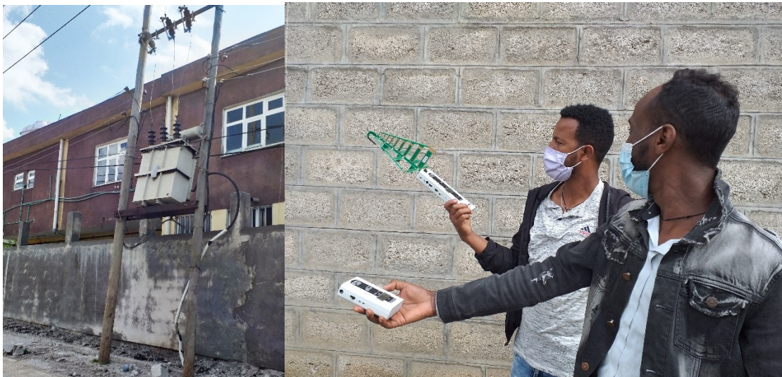
Figure 32: 630Kv transformer in Haile garment industry area (a) 630Kv transformer and (b) EF and MF recording on the site
