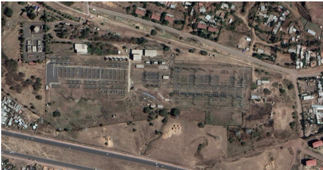
Figure 10: Aerial view of Kality I substation
