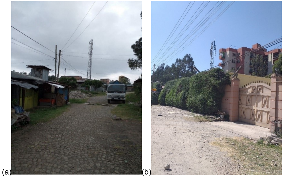
Figure 11: a) Cellphone tower in the middle of neighborhood and b) on the roof of a building Transformer positions in the neighborhood
