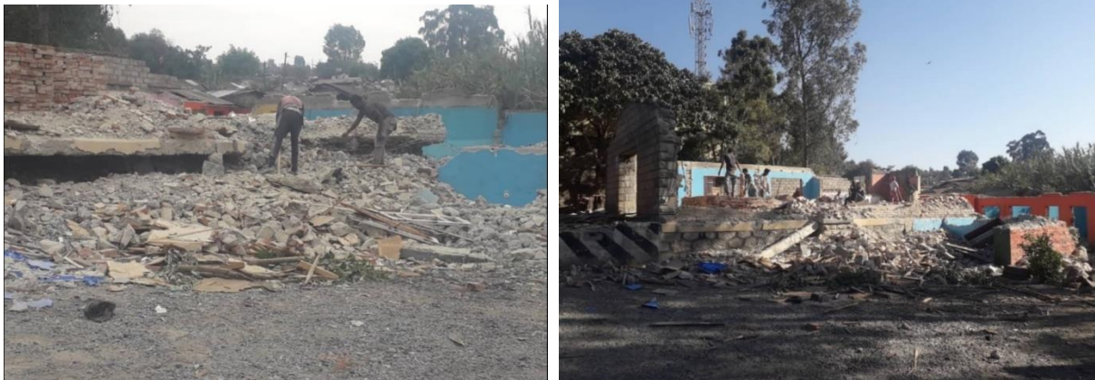
Fig. 4.12 (a) Manual demolition of existing structural elements, Jan. 2021 (Source: self-taken)
