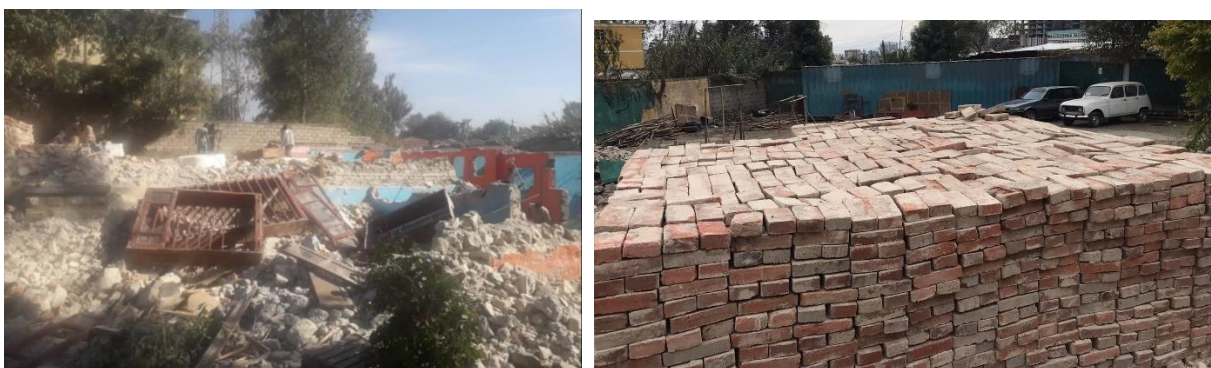
Fig. 4.12 (b) Material extraction for reuse, Jan. 2021 (Source: self-taken)
