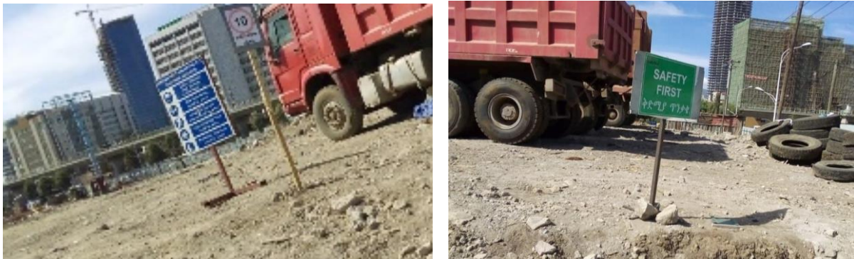
Fig. 4.15 Safety signage inside the site compound, Dec. 2020 (Source: self-taken)
