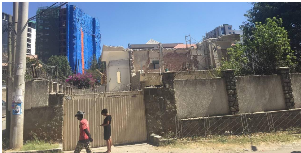
Fig. 4.14 Demolition of a residential building, Dec. 2020 (Source: self-taken)
