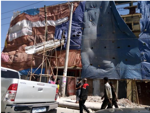
Fig. 4.13 Dust control mechanism, Dec. 2020 (Source: self-taken) (left), Demolition taking place, Dec. 2020 (Source: self-taken) (right)
