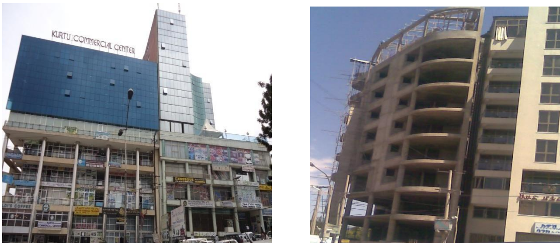
Figure 7: Sample adjacent building with different floor level. a. found at Habte Gorgis Dildy, Kirtu commercial center, b. found at Bole, K.Z Hotel, Addis Ababa.
