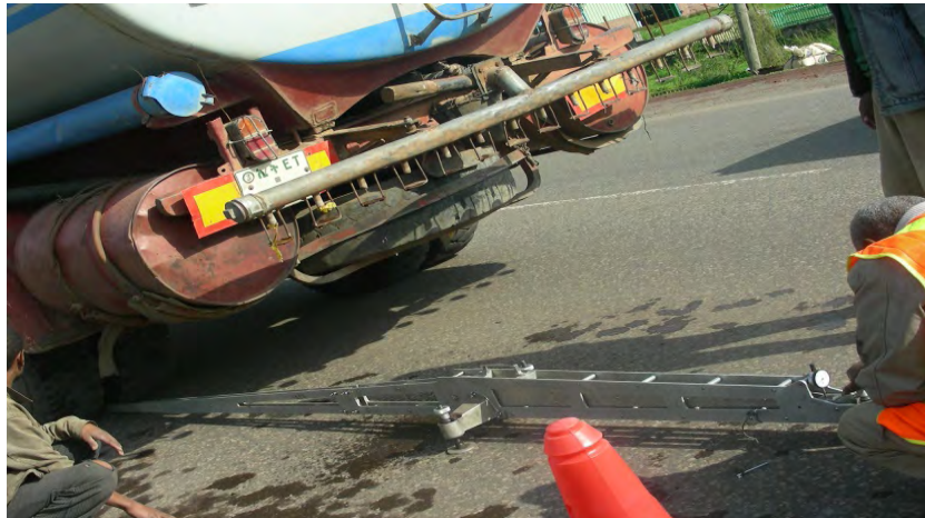
Figure 4-10: Benkelman Beam Deflection Measurement
