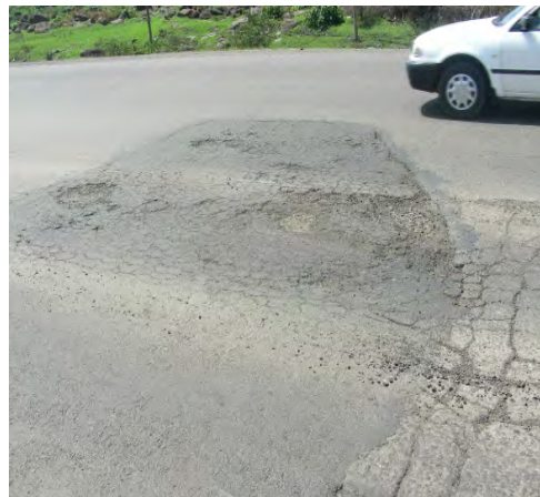
f) Repaired Section
