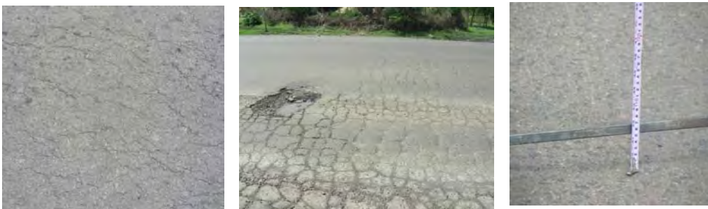
Photo 1.1 Existing condition of the pavement and measurement
