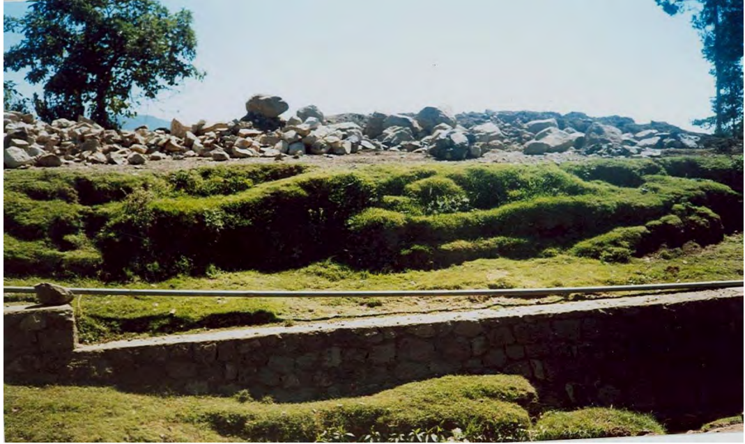
Figure 4.8 Exposed pipe in Font Nina spring development
