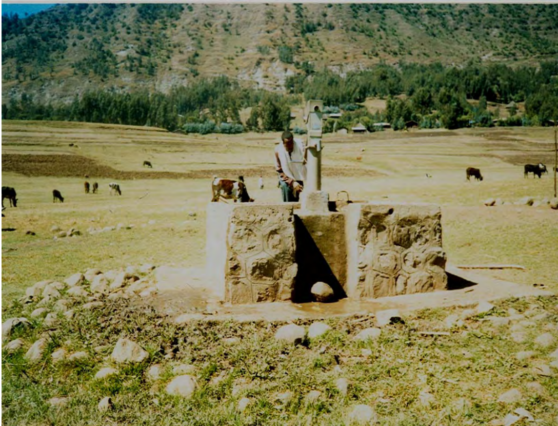
Figure 4.1 Hand dug well in Kelem Myda
