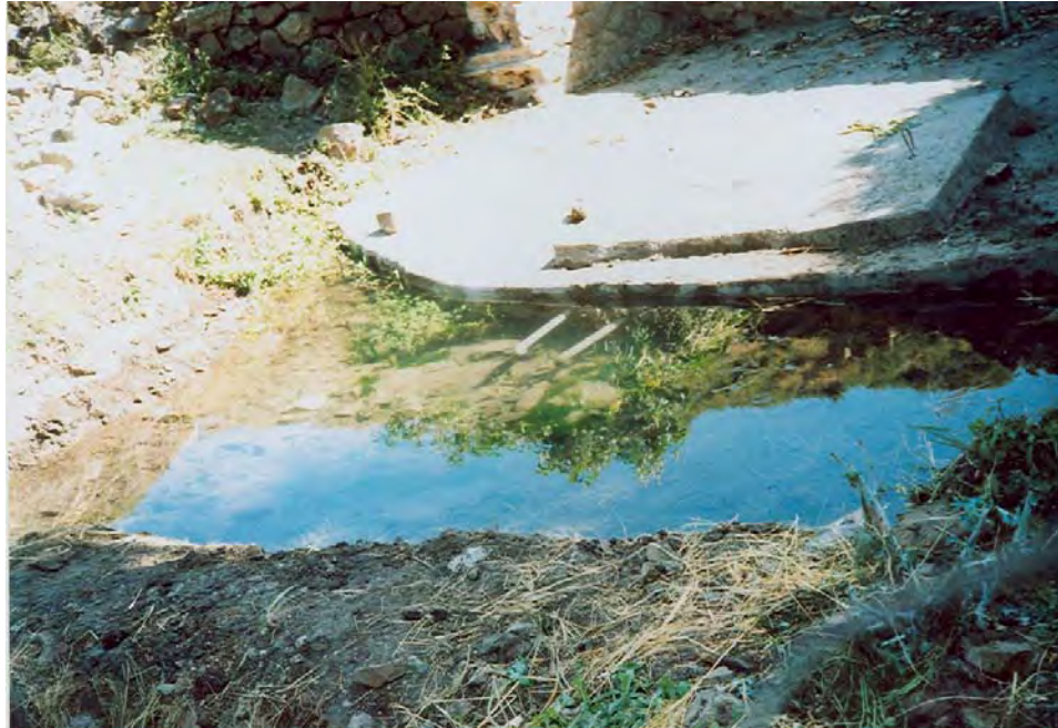
Figure 4.6 Improper spring tapping in Assa Erbat
