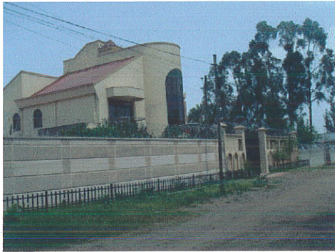
Figure 4.29 Neighboring Rented Residence
