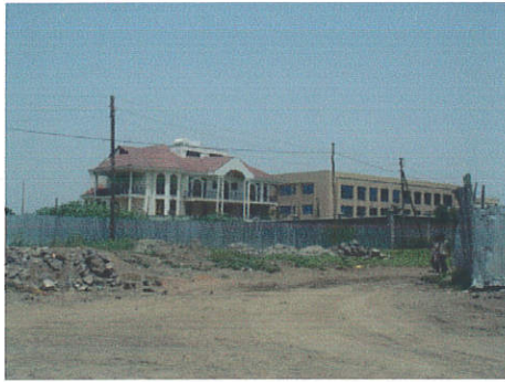
Figure 4.41 Office converted to Luxurious Residence
