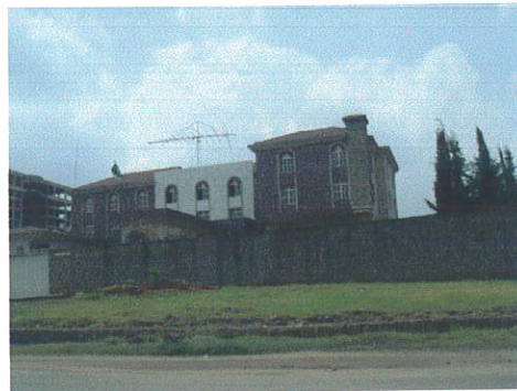
Figure 4.17 Algeria Embassy Chancery.
