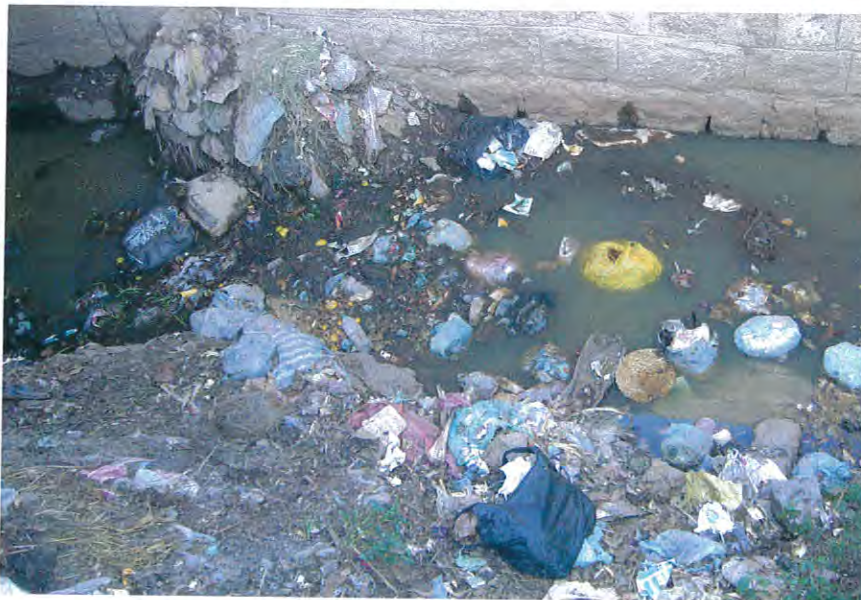
Figure 4.10: An Open Ditch Filled with Sewer and Plastic Bags, Possibly with Human Waste. (Tureta Sefer: 2007)
