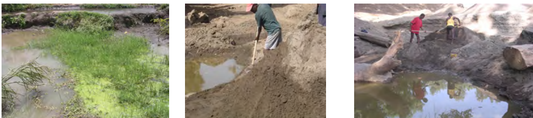
C. Canal leakage pool (left) and sand pools (right).
