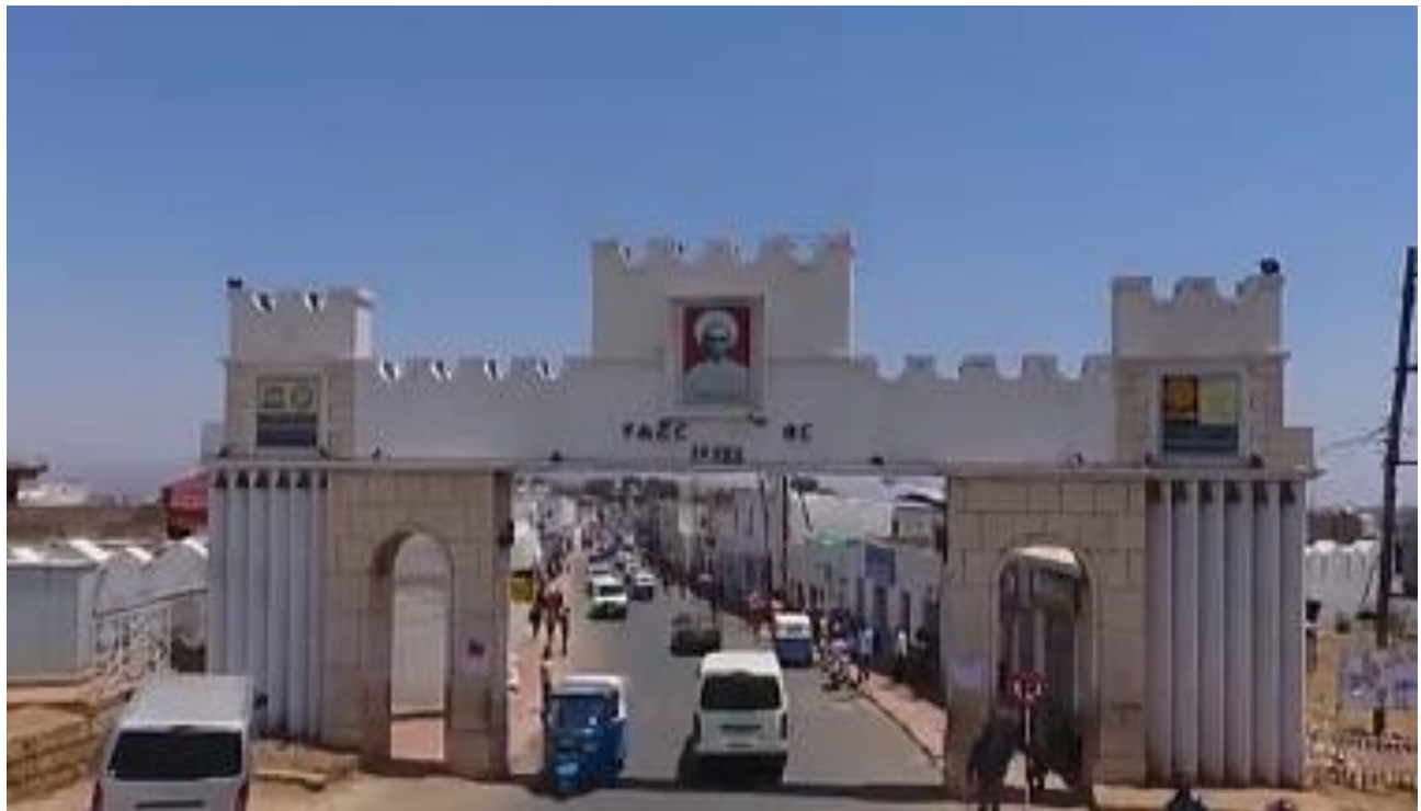
Figure 4: Harar Entrance of the Jegol wall 5
