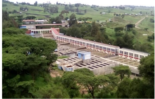
Figure 5. Legedadi water treatment plant
