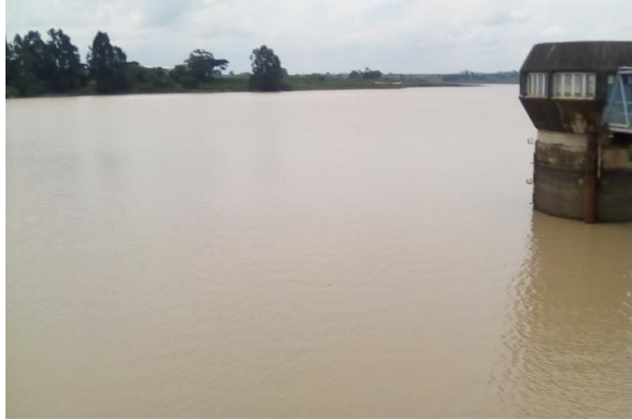
Figure 4. Legedadi water reservoir
