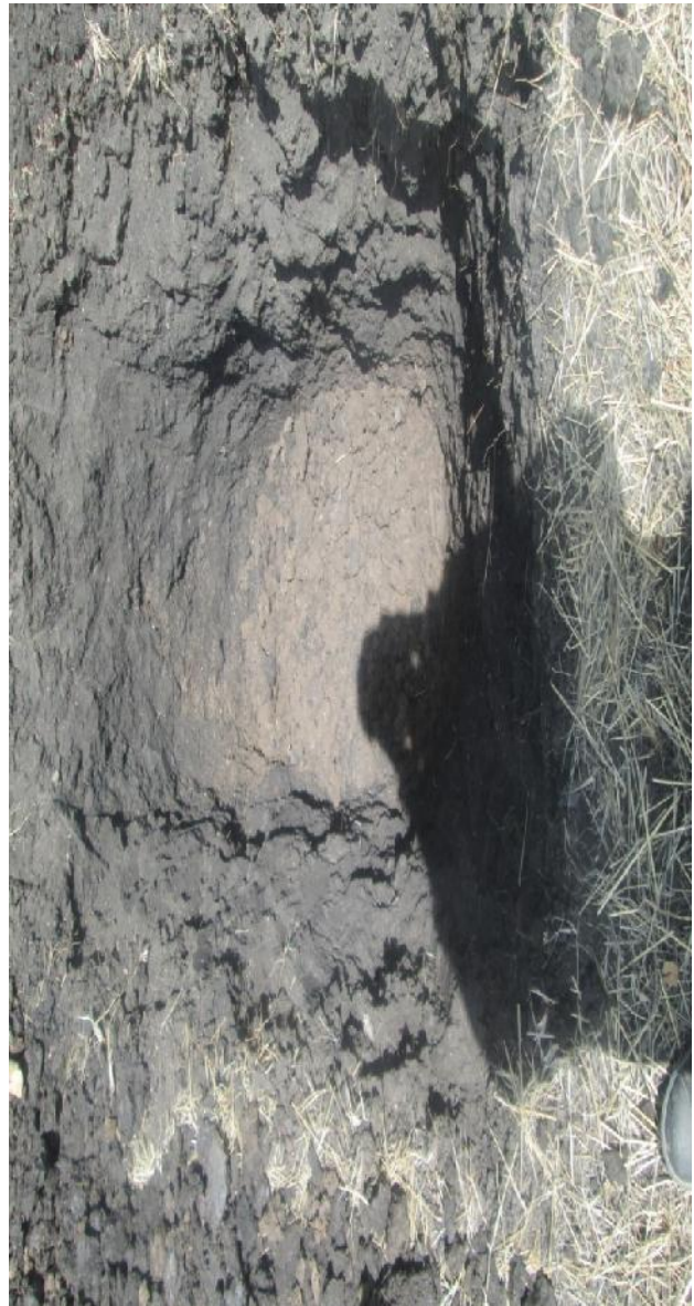
photo 7 Test pit taken for subgrade at 28 + 400
