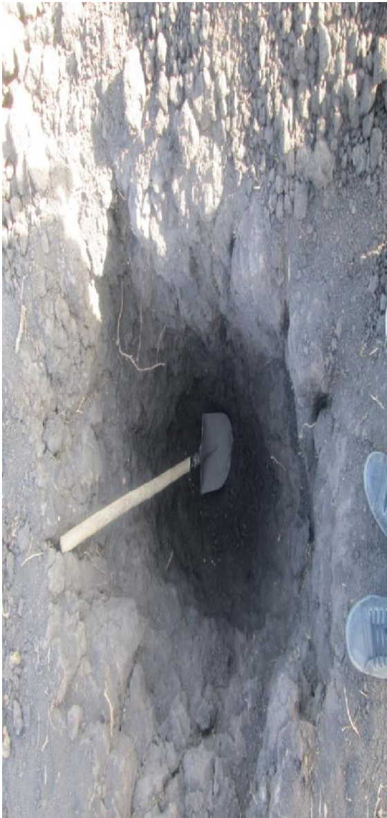
Photo 6 Test pit taken at station 9 + 656
