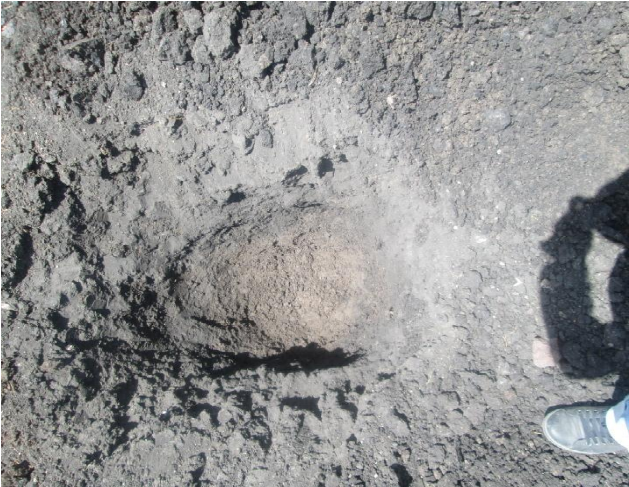
Photo 5 Test pit taken for subgrade at station 10 + 080
